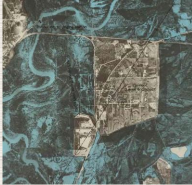
Flowood levee built 1935 -1940
