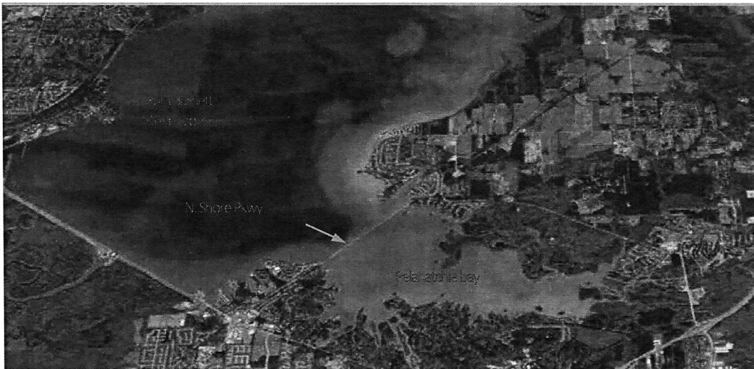
Figure 4. Aerial visual (2020) of sedimentation in Pelahatchie Bay from construction activities.
