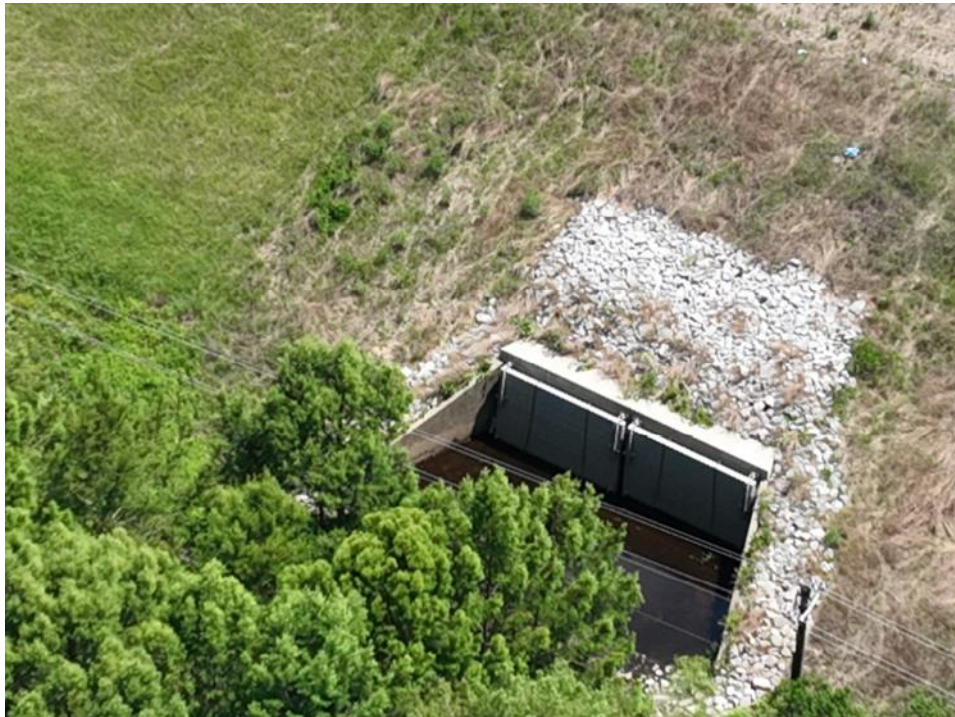
Figure 1-39 Example of Gates added to existing structures.
