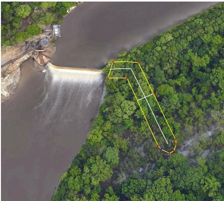
Figure 2-13. Stone Placement East Bank to protect the Fewell Treatment Plant Weir
