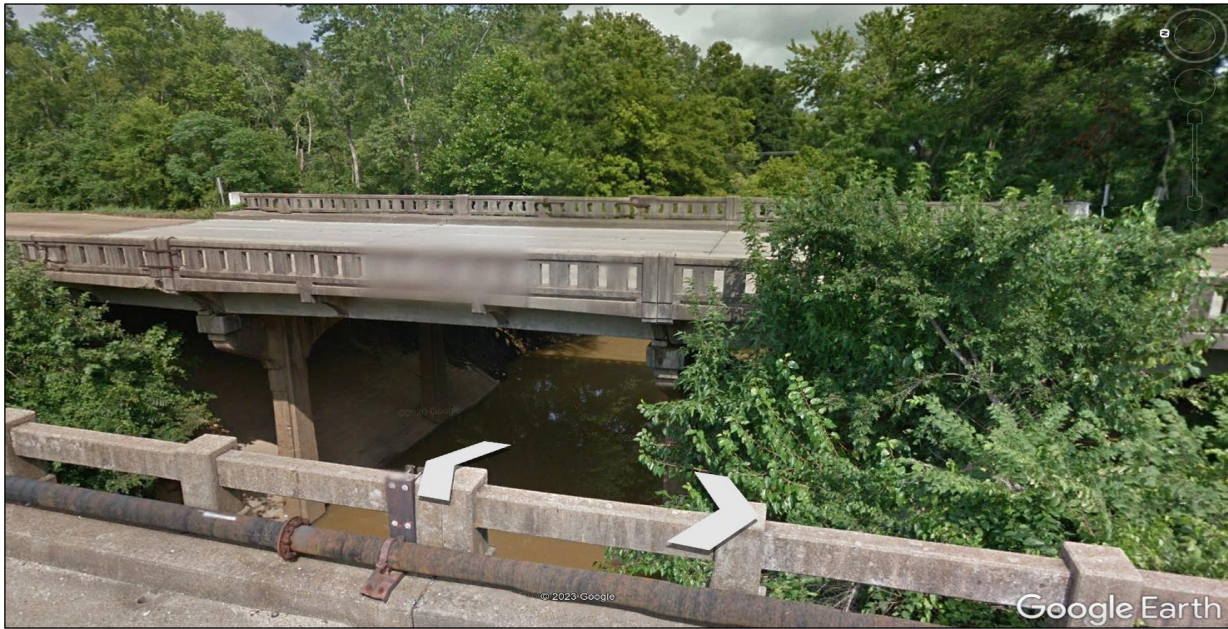
Figure E3-9 Town Creek at an Abandoned Road/Bridge Just Upstream of State Street, Looking Downstream at State Street
