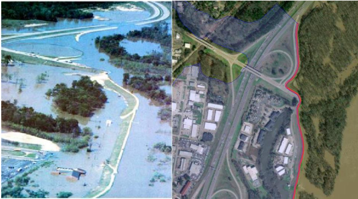
Figure 2-7: 1984 Levee Extension to Prevent Flanking
