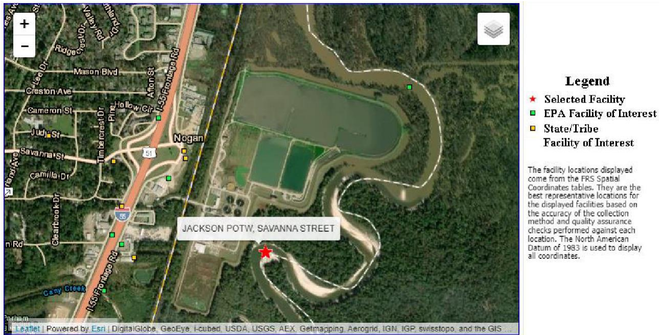
Figure 2-3: Savannah Wastewater Treatment Plant
