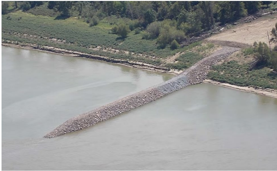
Figure A-156. Typical Stone Dike Construction with Dig-In
