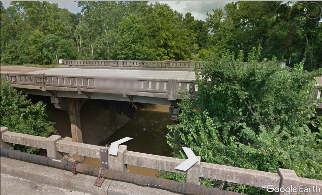
Figure E3-9 Town Creek at an Abandoned Road/Bridge Just Upstream of State Street, Looking Downstream at State Street
