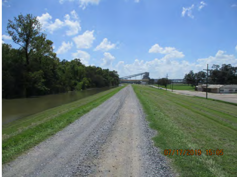
Figure 2: West facing picture near the center of the alignment, Saint James Parish, Louisiana.
