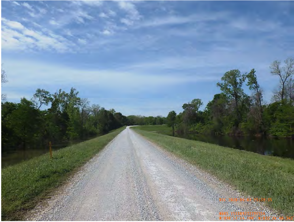
Figure 2: Southwest facing picture of the proposed levee enlargement, Issaquena County, Mississippi.
