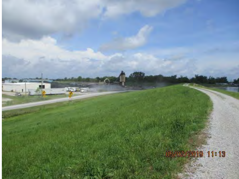
Figure 2: Northwest facing picture near the northern end of the alignment, West Baton Rouge Parish, Louisiana.
