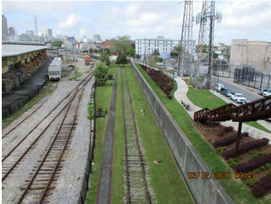
Figure 2: West facing picture near the center of the alignment, Orleans Parish, Louisiana.
