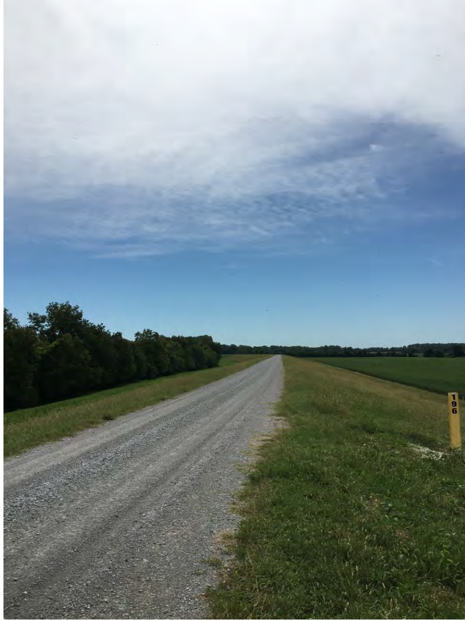
Figure 2: Representative photograph of the site, facing S (downstream) along the mainline Mississippi River Levee crown near Levee Mile Post 196/197 within the proposed project boundaries.
