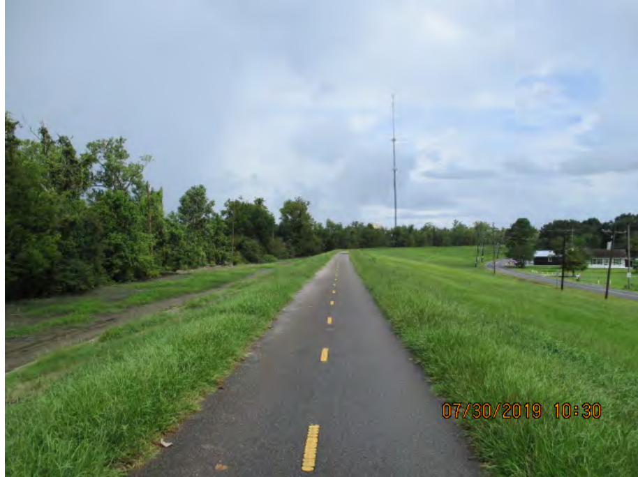
Figure 2: Northwest facing picture near the center of the alignment, Saint John the Baptist Parish, Louisiana.
