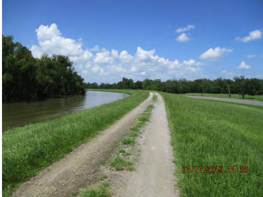
Figure 2: Northeast facing picture near the center of the alignment, Ascension Parish, Louisiana.
