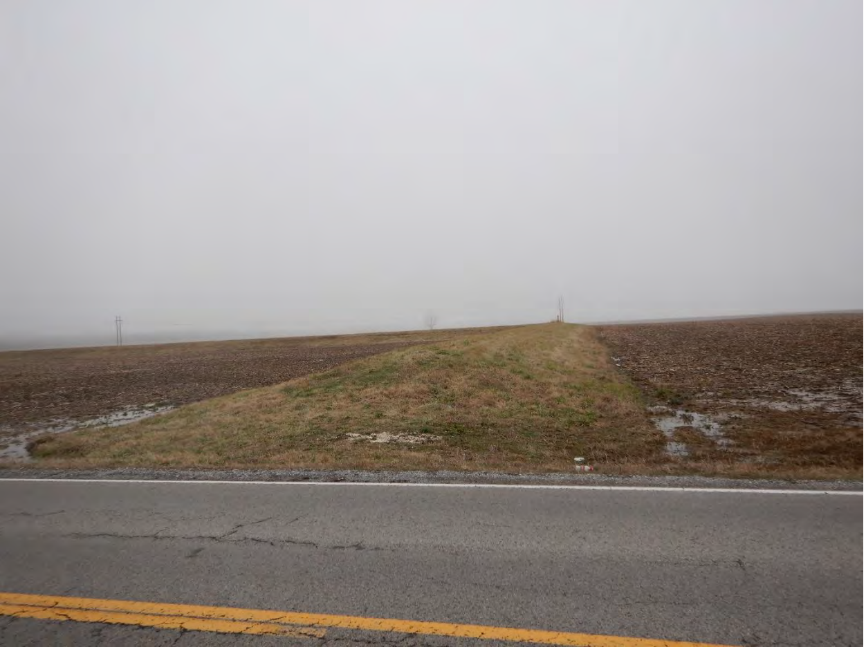
Figure 2: Photograph representative of the project area, facing the levee (north) from Illinois Highway 8, at the far upstream limits of the project area where the levee ties into high ground.
