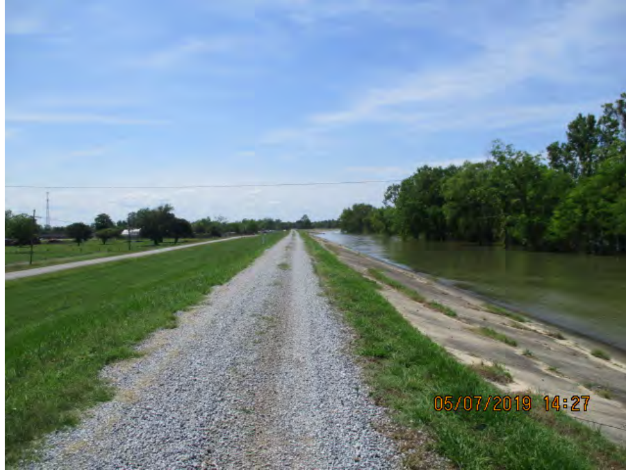
Figure 2: Northwest facing picture near the center of the alignment, Iberville Parish, Louisiana.
