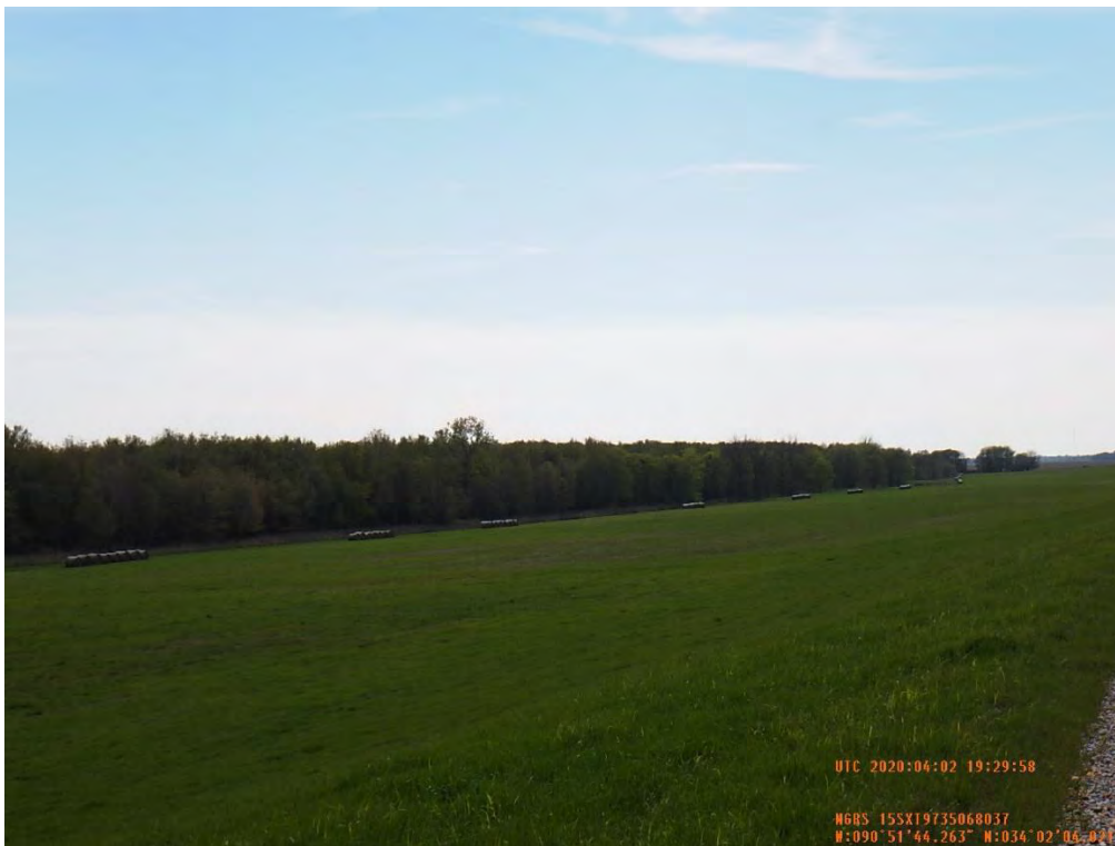
Figure 3: East facing picture of the proposed seepage berm location, Bolivar County, Mississippi.
