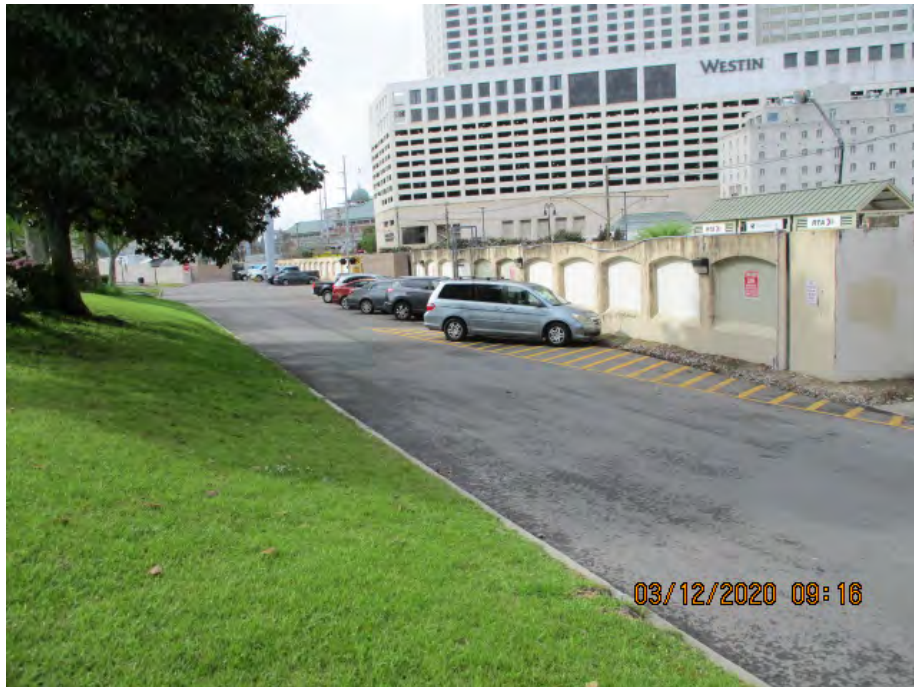
Figure 2: South facing picture near the center of the alignment, Orleans Parish, Louisiana.
