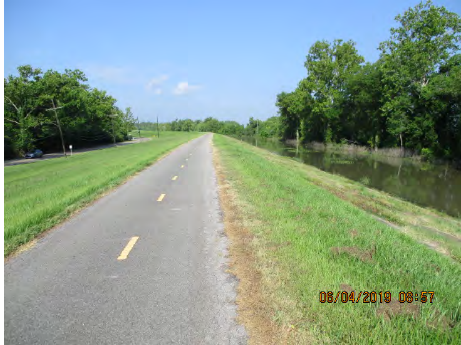
Figure 2: Southwest facing picture near the center of the alignment, Saint Charles Parish, Louisiana.
