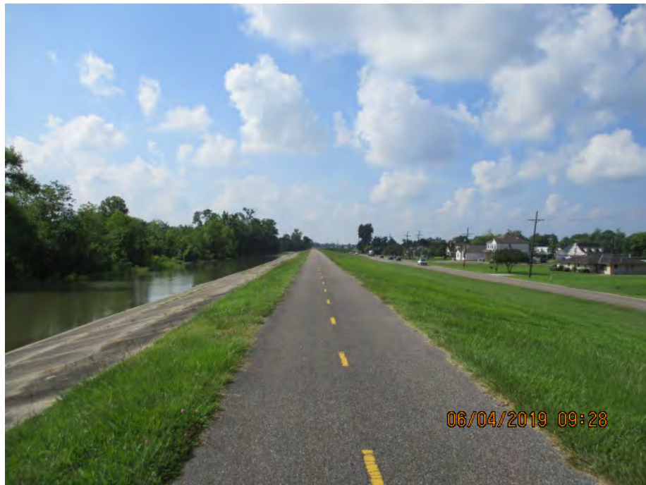
Figure 3: Southeast facing picture near the center of the alignment, Jefferson Parish, Louisiana.
