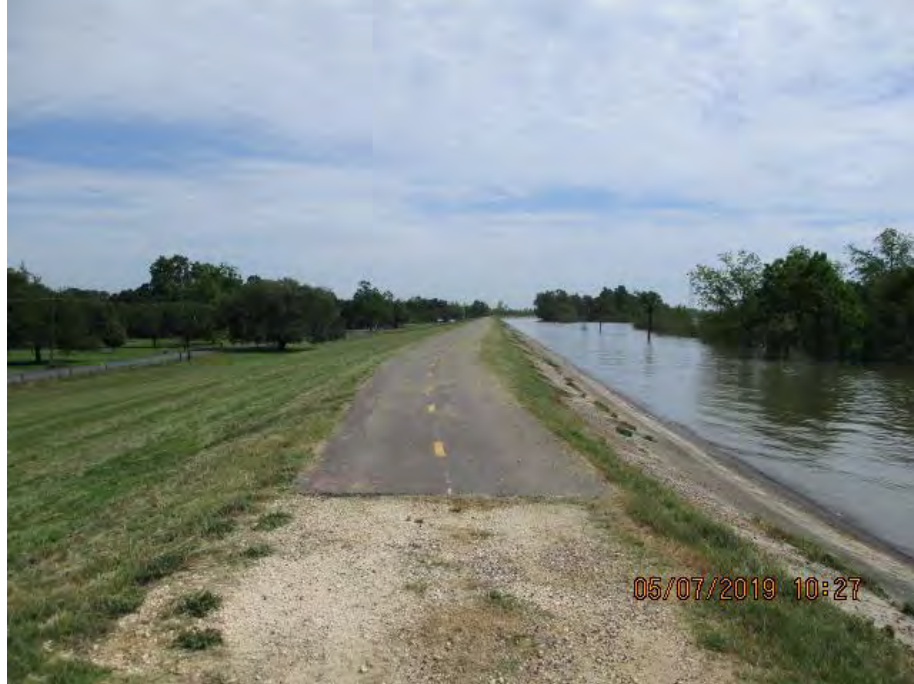
Figure 2: North facing picture near the center of the alignment, West Baton Rouge Parish, Louisiana.
