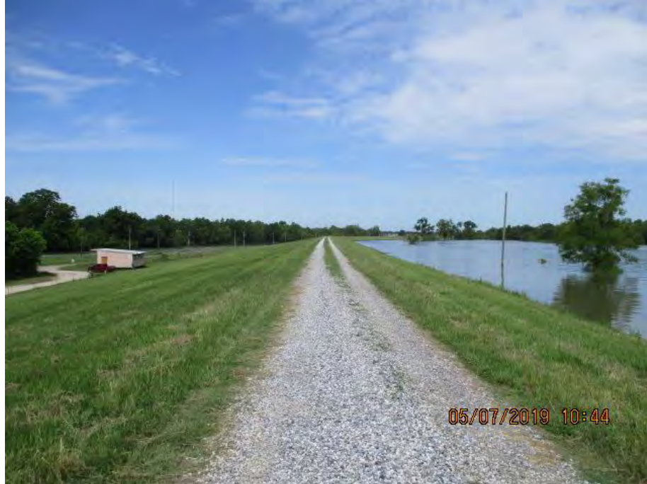
Figure 2: Northwest facing picture near the center of the alignment, East Baton Rouge and Iberville Parishes, Louisiana.
