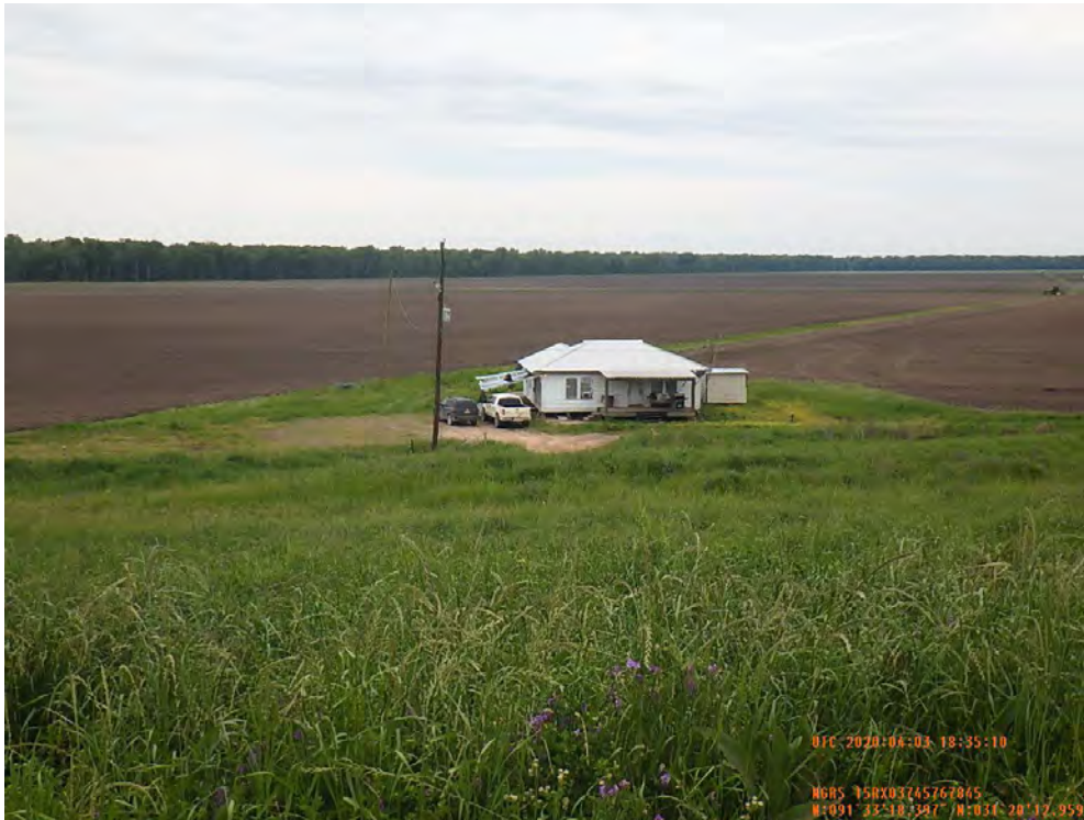
Figure 4: West facing picture for the proposed location of seepage berm with residential structure, Concordia Parish, Louisiana.
