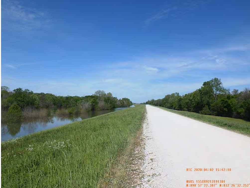
Figure 4: Northwest facing picture of the proposed levee enlargement, Issaquena County, Mississippi.
