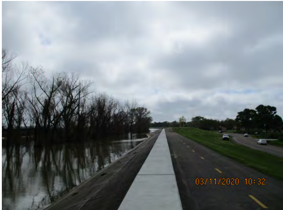
Figure 3: South facing picture near the center of the Waggaman Floodwall alignment, Jefferson Parish, Louisiana.
