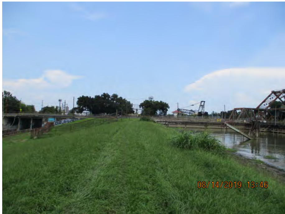
Figure 5: North facing picture near the center of the alignment_on west side of IHNC Forebay, Orleans Parish, Louisiana.
