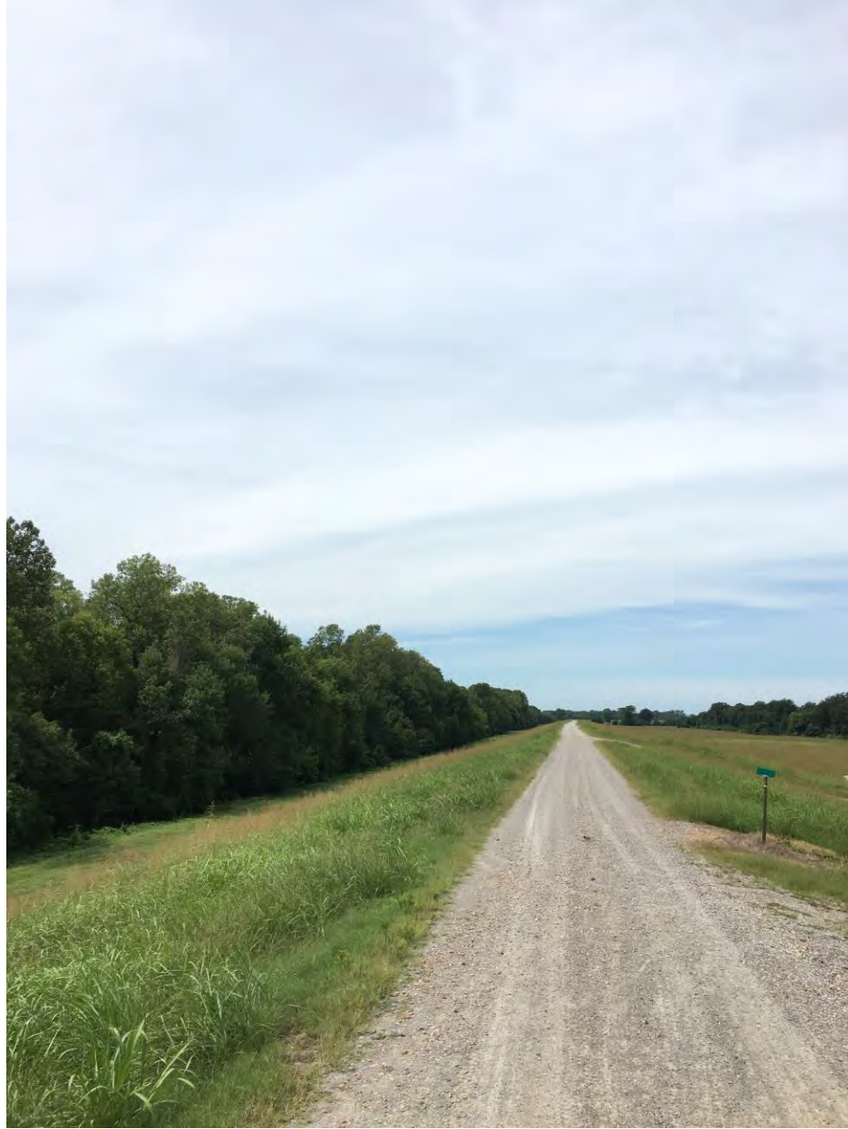
Figure 2: Facing W (downstream) along the mainline Mississippi River Levee crown near Levee Mile Post 200/201 within the proposed project boundaries.
