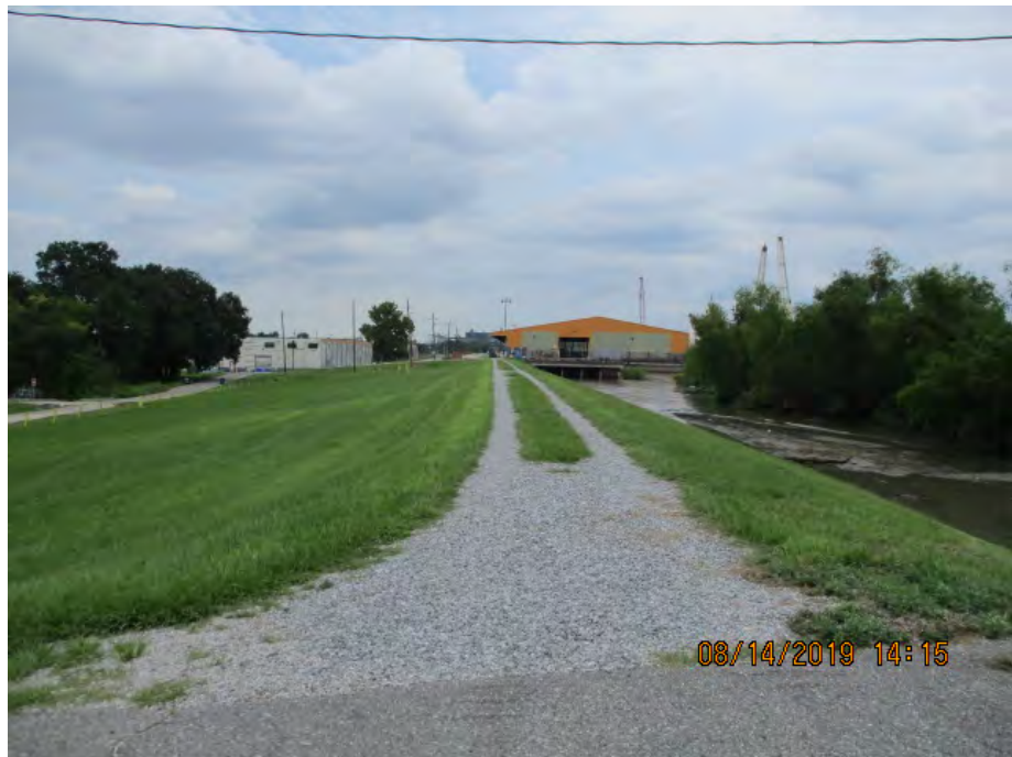
Figure 3: East facing picture near the center of the alignment, Orleans Parish, Louisiana.
