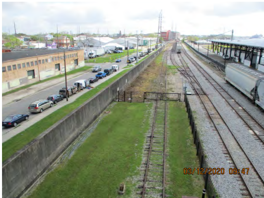
Figure 3: East facing picture near the center of the alignment, Orleans Parish, Louisiana.
