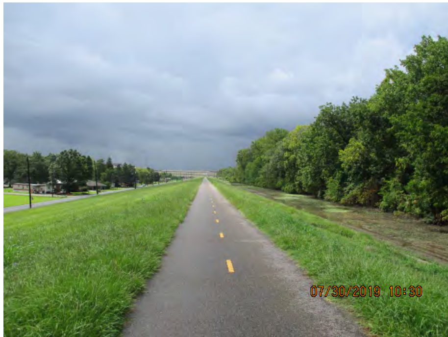
Figure 3: Southeast facing picture near the center of the alignment, Saint John the Baptist Parish, Louisiana.
