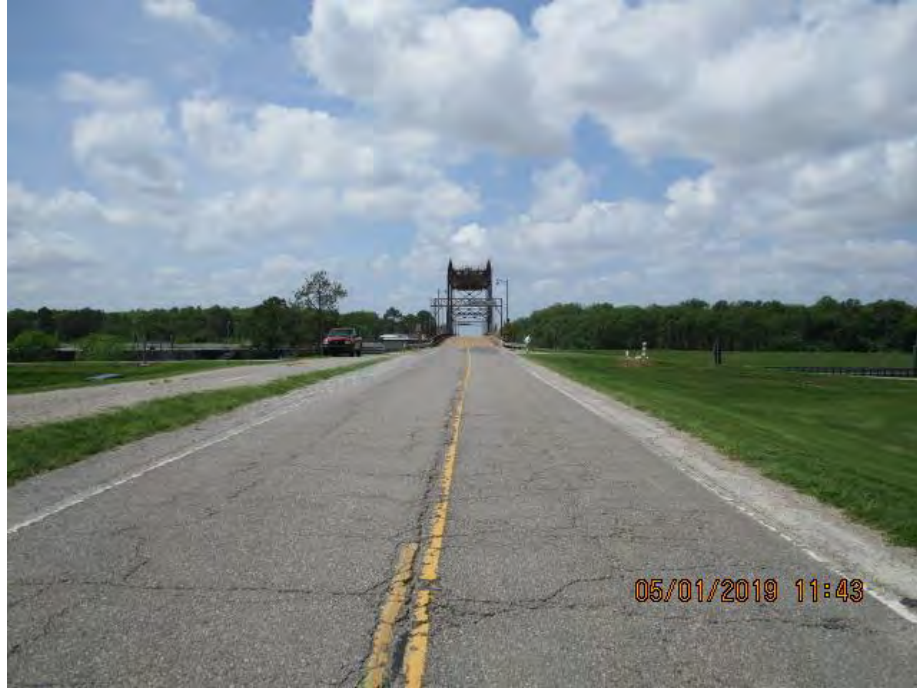
Figure 2: Southwest facing picture near the center of the alignment, Pointe Coupee Parish, Louisiana.
