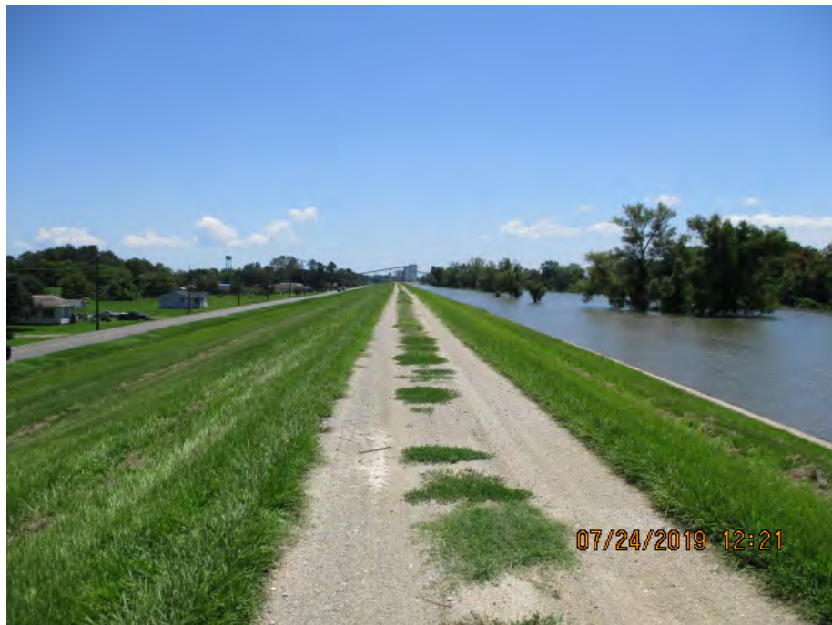
Figure 3: East facing picture near the center of the alignment, Saint James Parish, Louisiana.
