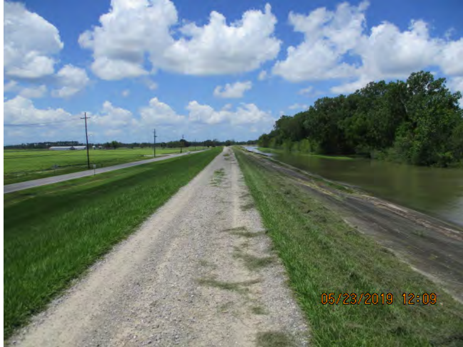
Figure 2: Southwest facing picture near the center of the alignment, Saint John the Baptist Parish, Louisiana.
