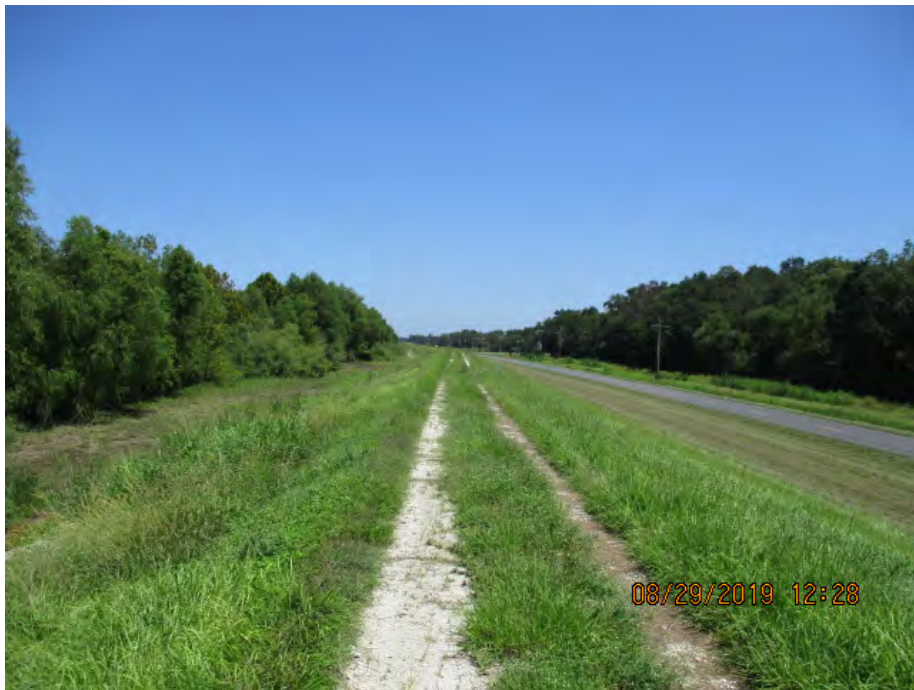
Figure 4: North facing picture near the center of the alignment, Plaquemines Parish, Louisiana.
