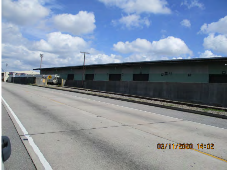
Figure 2: West facing picture near the center of the alignment, Orleans Parish, Louisiana.
