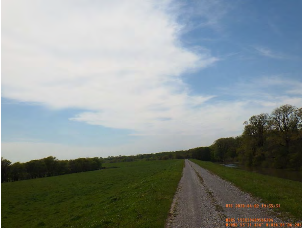
Figure 4: East facing picture of the proposed seepage berm location, Bolivar County, Mississippi.
