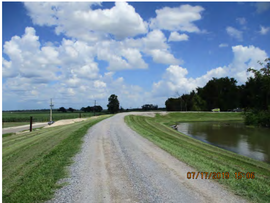
Figure 3: East facing picture near the center of the alignment, Saint James Parish, Louisiana.
