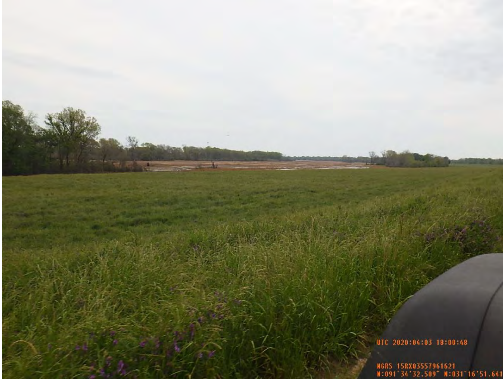
Figure 2: East facing picture for the proposed location of relief wells, Concordia Parish, Louisiana.
