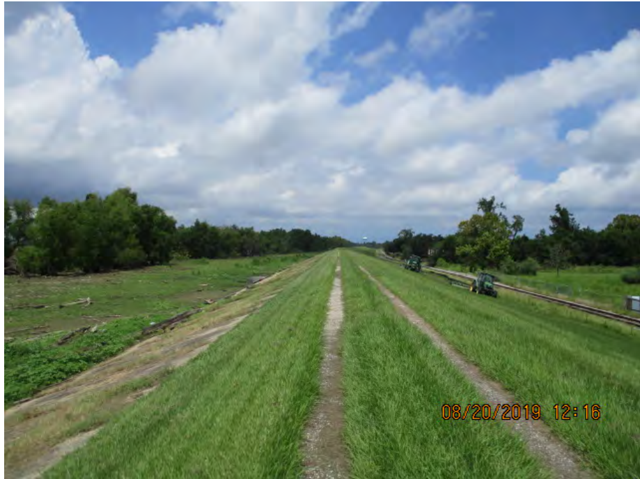
Figure 2: Northwest facing picture near west end of the alignment, St. Bernard Parish, Louisiana.
