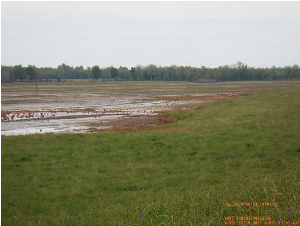
Figure 5: East facing picture of existing relief well in the proposed location for future relief wells, Concordia Parish, Louisiana.
