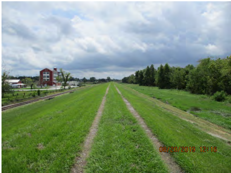
Figure 3: Southeast facing picture near west end of the alignment, St. Bernard Parish, Louisiana.
