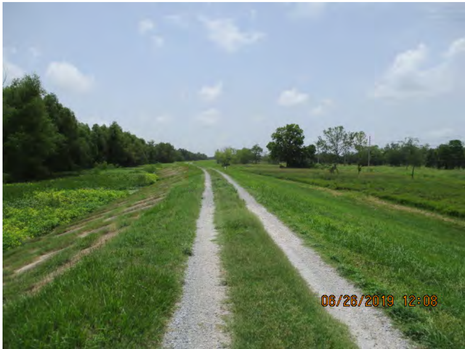
Figure 3: Southeast facing picture near the center of the alignment, Plaquemines Parish, Louisiana.
