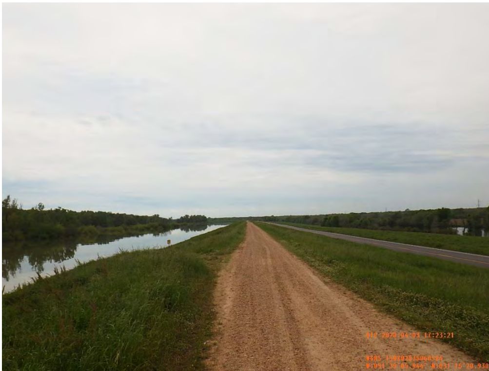
Figure 3: Southwest facing picture from the levee crown for the proposed enlargement, Concordia Parish, Louisiana.
