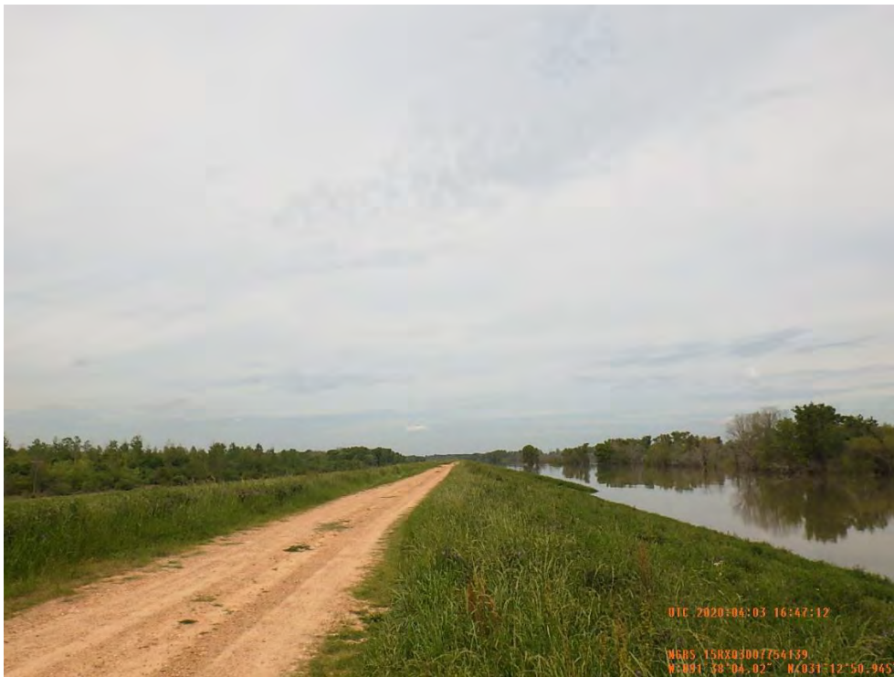
Figure 3: Northwest facing picture from the levee crown for the proposed enlargement, Concordia Parish, Louisiana.
