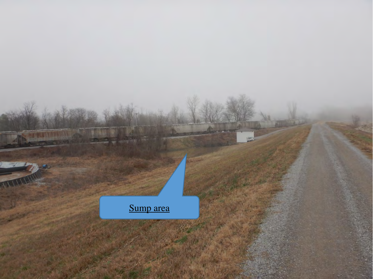
Figure 2: Photograph representative of the project area, facing the sump area (north) along the levee.
