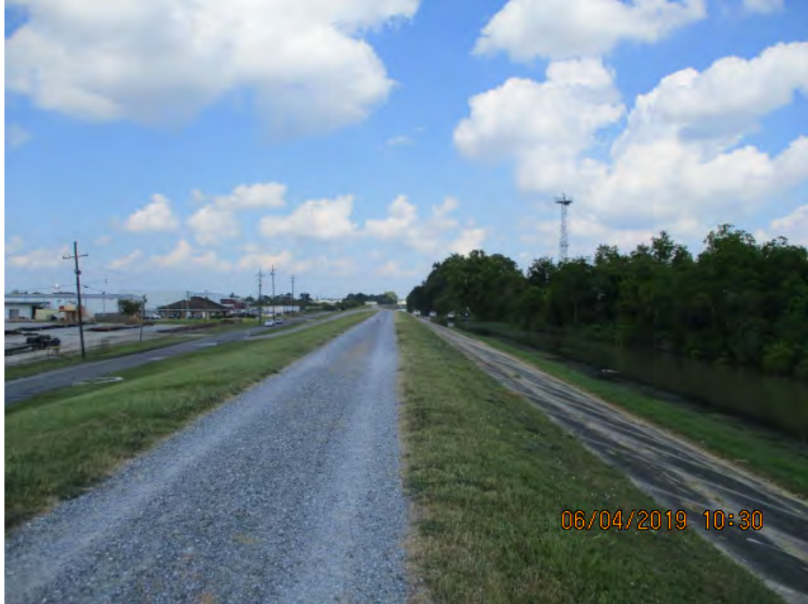
Figure 2: West facing picture near the center of the alignment, Jefferson Parish, Louisiana.
