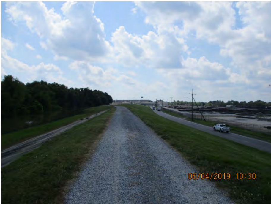
Figure 3: East facing picture near the center of the alignment, Jefferson Parish, Louisiana.
