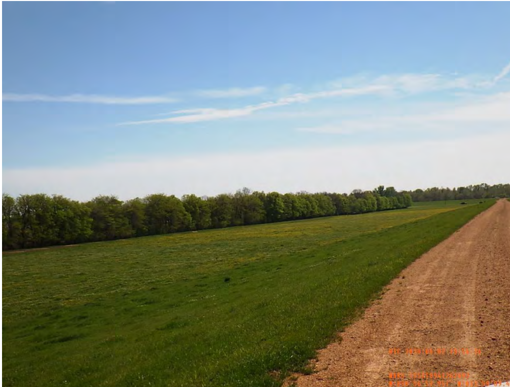
Figure 7: East facing picture of the proposed seepage berm location, Bolivar County, Mississippi.
