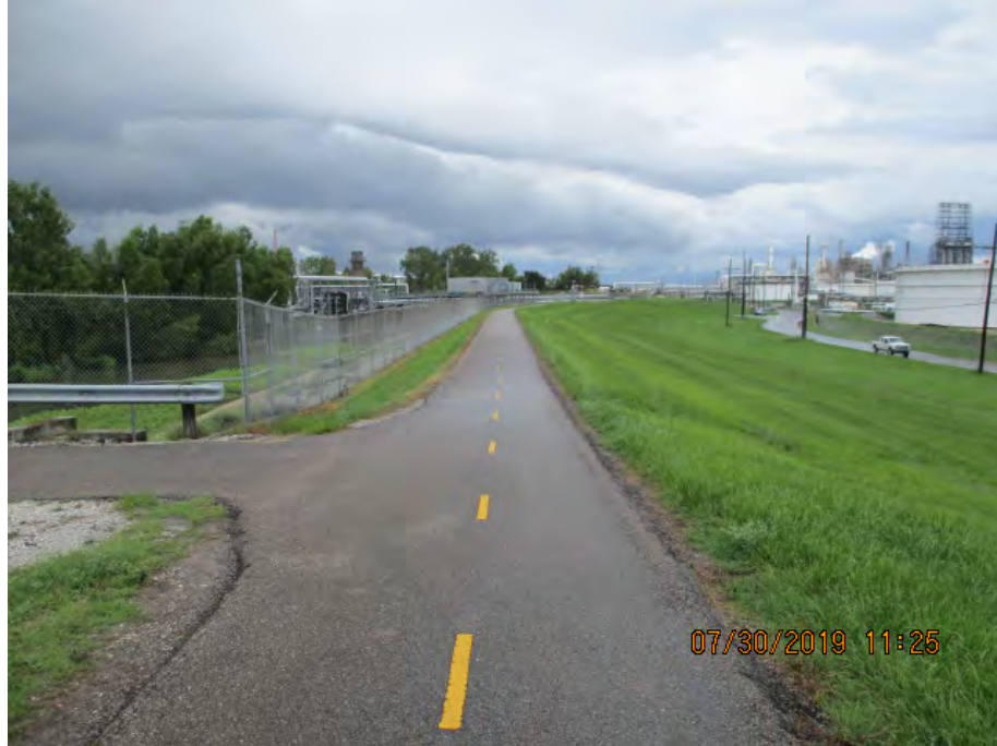
Figure 2: Northwest facing picture near the center of the alignment, Saint Charles Parish, Louisiana.
