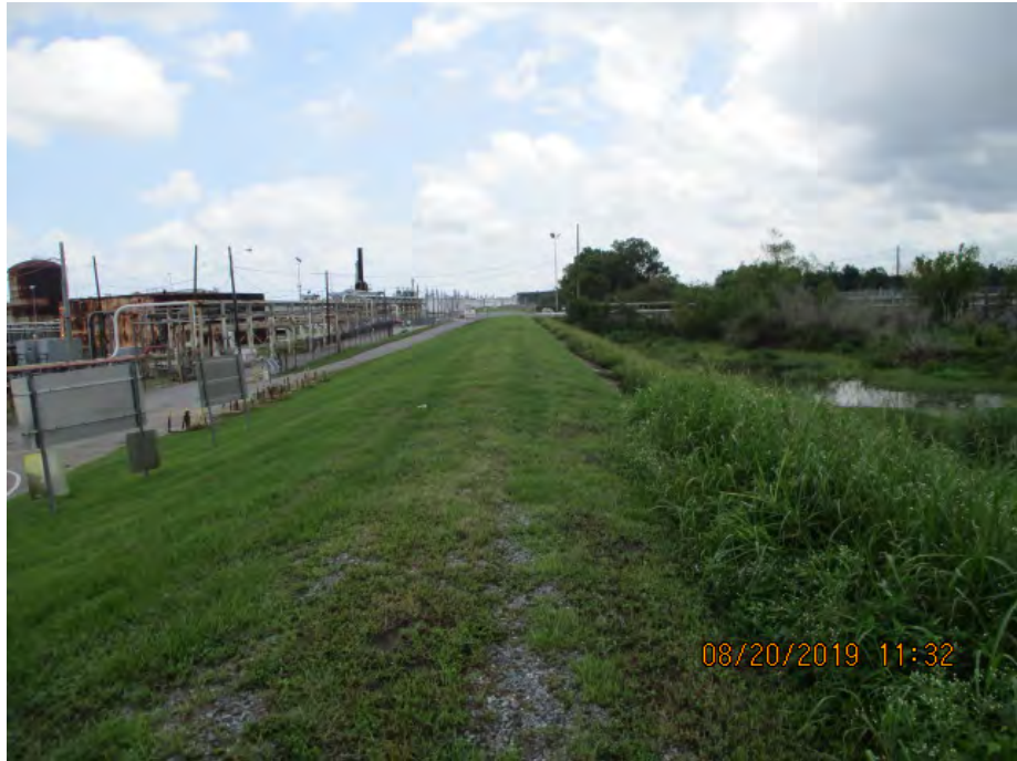
Figure 4: West facing picture near center of the alignment, St. Bernard Parish, Louisiana.
