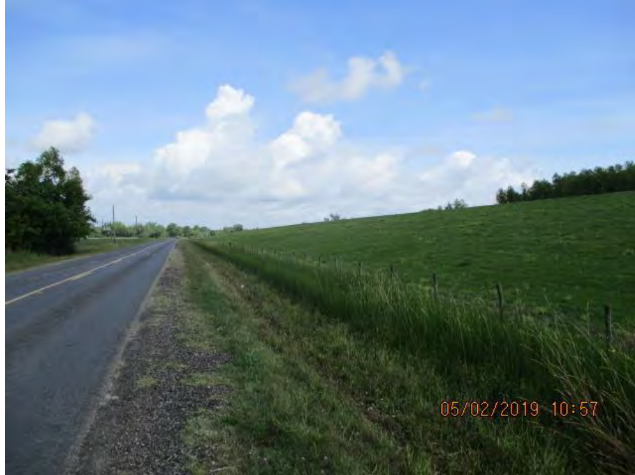
Figure 2: Northwest facing picture near the center of the alignment, West Baton Rouge Parish, Louisiana.
