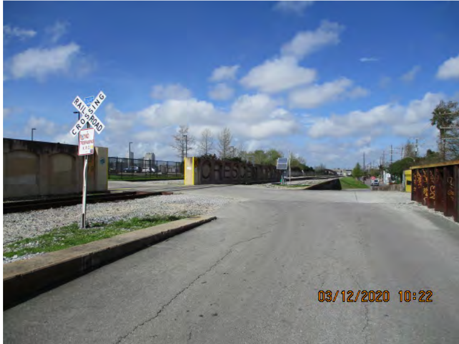
Figure 2: West facing picture near the center of the alignment, Orleans Parish, Louisiana.
