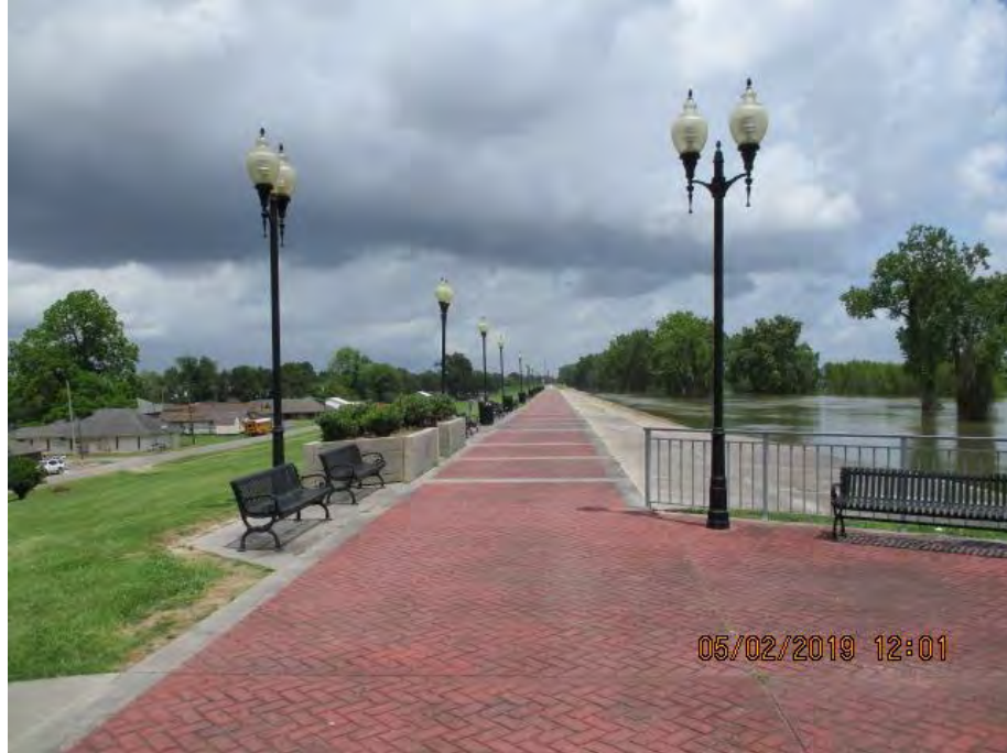
Figure 6: North facing picture near the southern end of the alignment, West Baton Rouge Parish, Louisiana.
