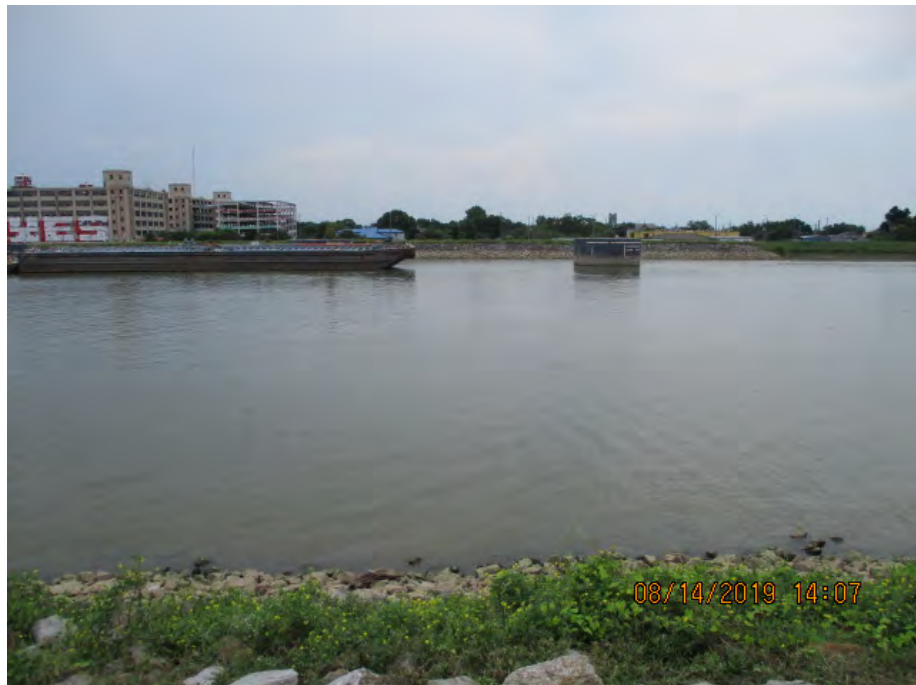
Figure 7: North facing picture near the center of the alignment on east side of IHNC Forebay, Orleans Parish, Louisiana.
