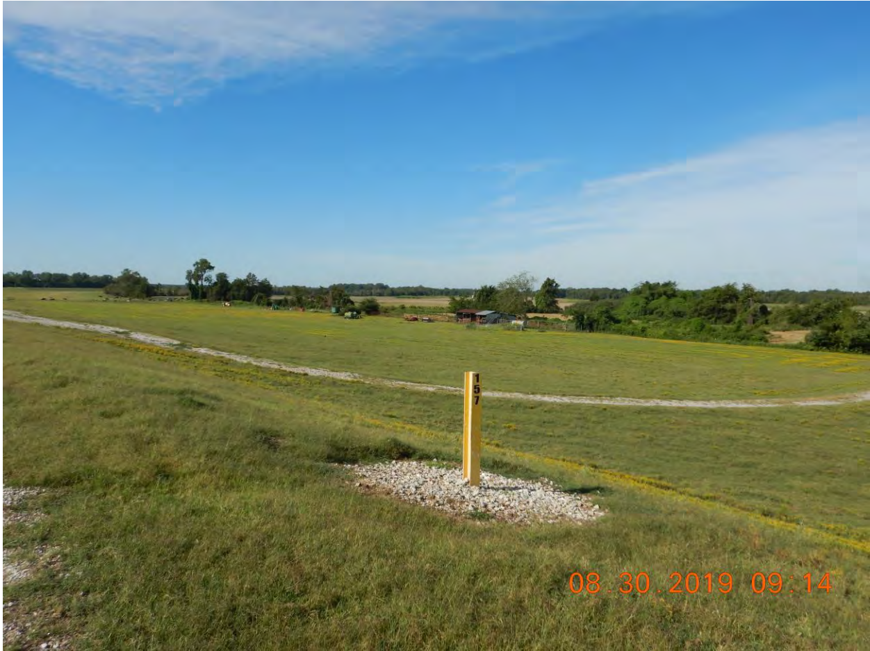
Figure 2: Representative photograph of the site, facing SW (downstream) towards the mainline Mississippi River Levee landside toe at Levee Mile Post 157/158 within the proposed project boundaries; note the farm operations and above ground storage tank in the distance.
