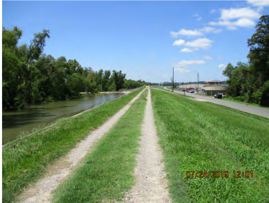
Figure 2: Southwest facing picture near the center of the alignment, Saint James Parish, Louisiana.
