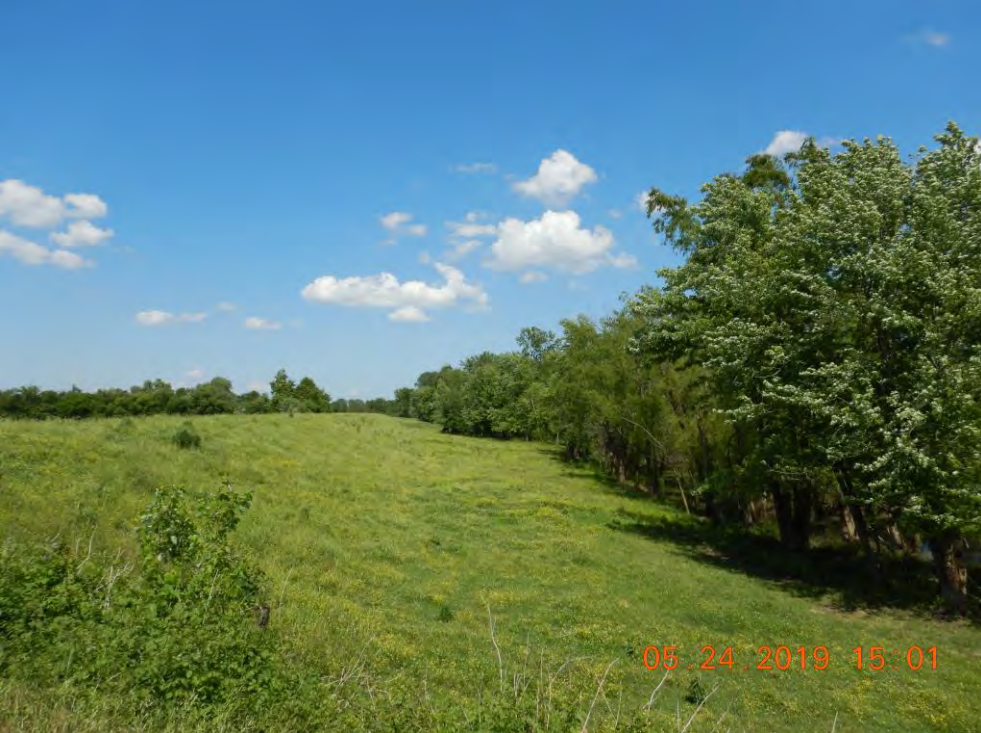
Figure 2: Representative photograph of the project area, facing upstream (north) along the riverside of the setback levee toe, near Missouri Highway 77, within the project area.
