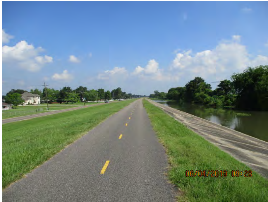
Figure 2: Northwest facing picture near the center of the alignment, Jefferson Parish, Louisiana.
