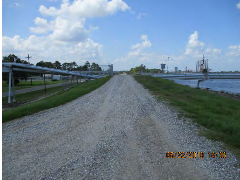
Figure 2: North facing picture near the center of the alignment, Saint James Parish, Louisiana.
