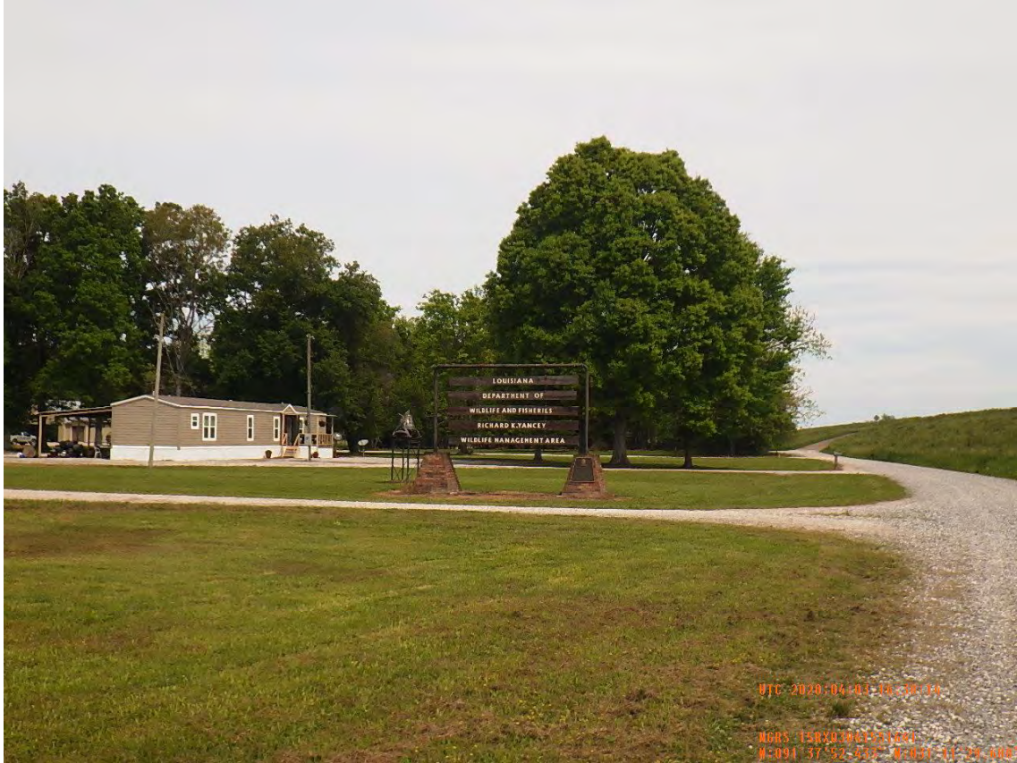
Figure 3: Northwest facing picture of levee toe for proposed seepage berm in front of the Richard K. Yancey - Wildlife Management Area Office, Concordia Parish, Louisiana.
