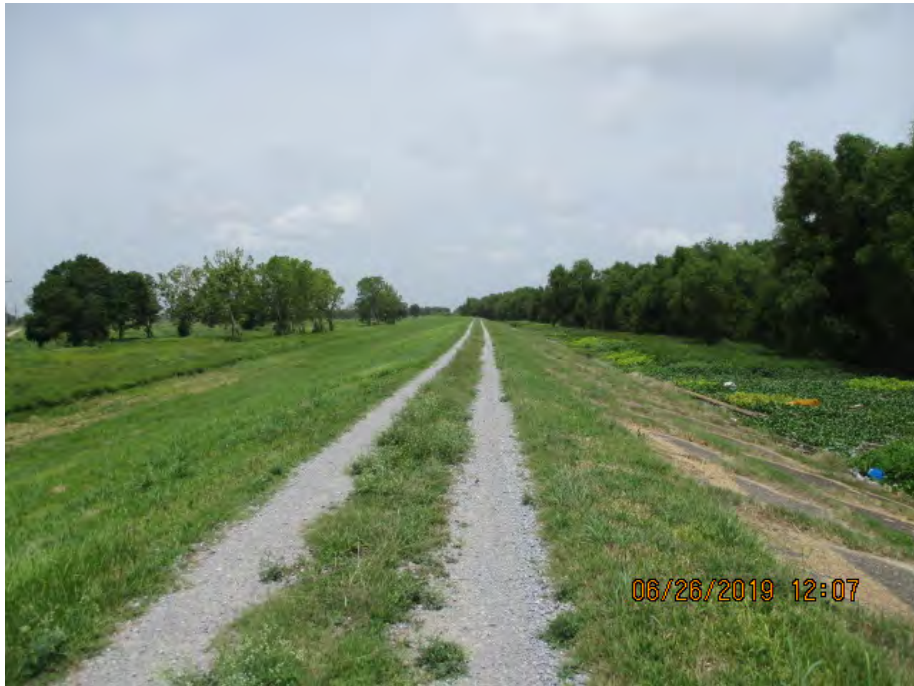
Figure 2: Northwest facing picture near the center of the alignment, Plaquemines Parish, Louisiana.
