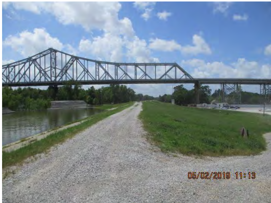
Figure 3: South facing picture near the northern end of the alignment, West Baton Rouge Parish, Louisiana.
