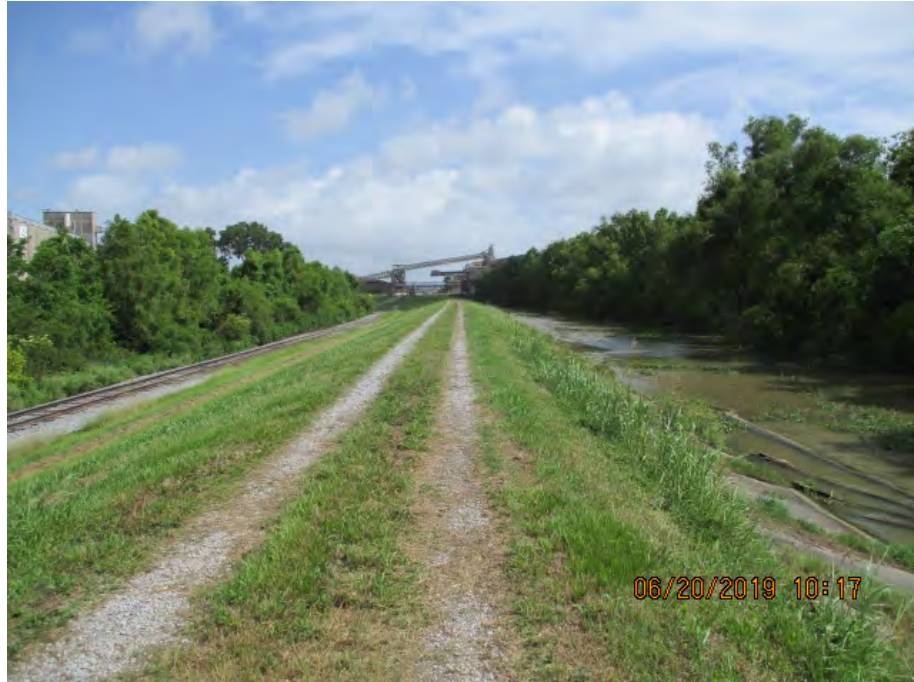
Figure 2: North facing picture near the center of the alignment, Plaquemines Parish, Louisiana.
