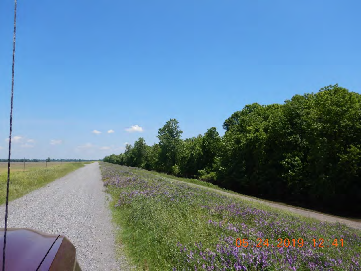
Figure 2: Representative photograph of the project area, facing upstream (north) along the frontline levee, near Lat. 36.619750, Long. -89.384111, within the project area.
