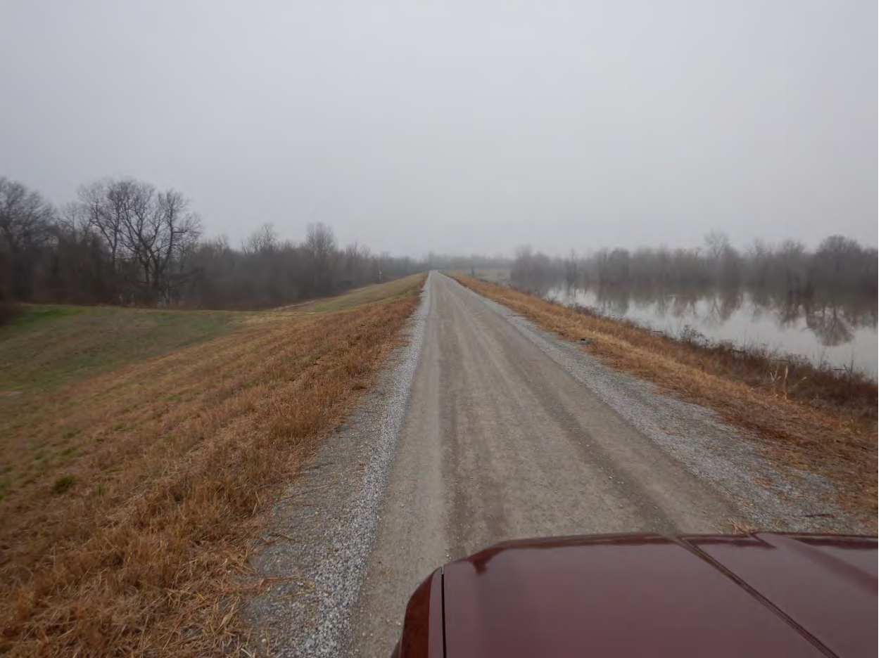
Figure 2: Photograph representative of the project area, facing upstream (north) along the levee within the downstream end of the project footprint.
