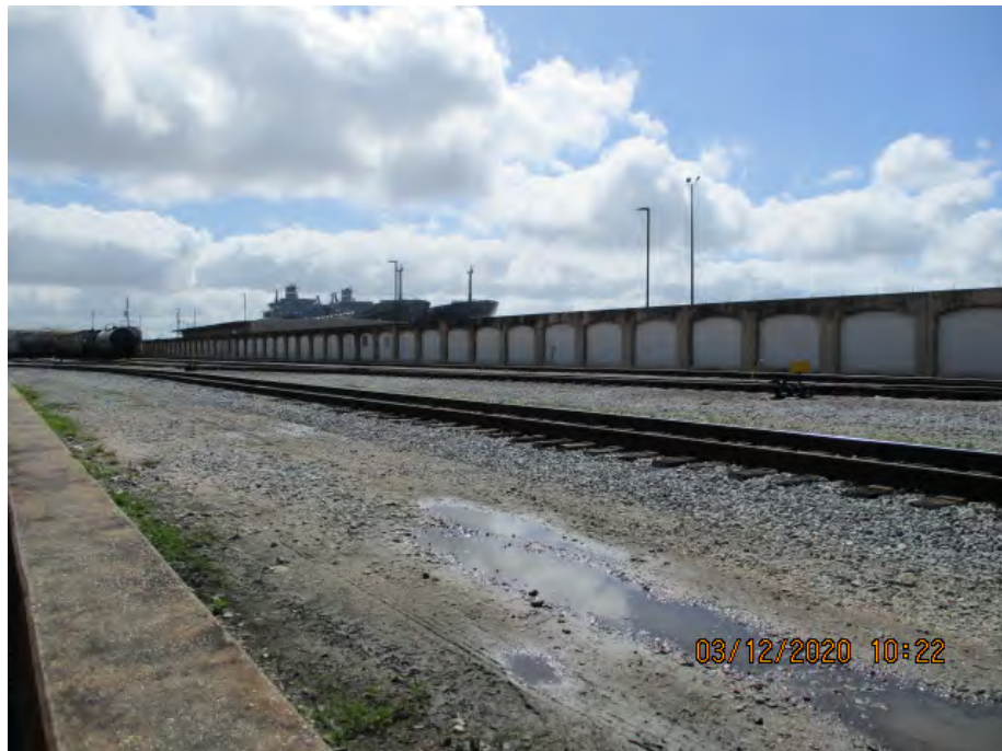
Figure 3: East facing picture near the center of the alignment, Orleans Parish, Louisiana.
