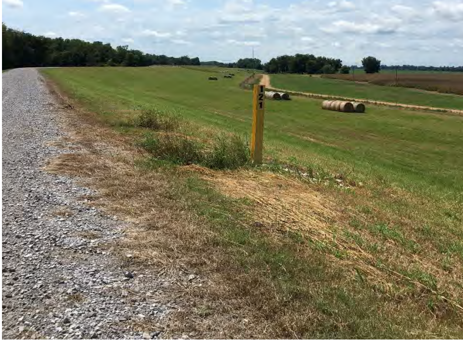
Figure 2: Representative photograph of the project area, facing downstream at Levee Station 121.
