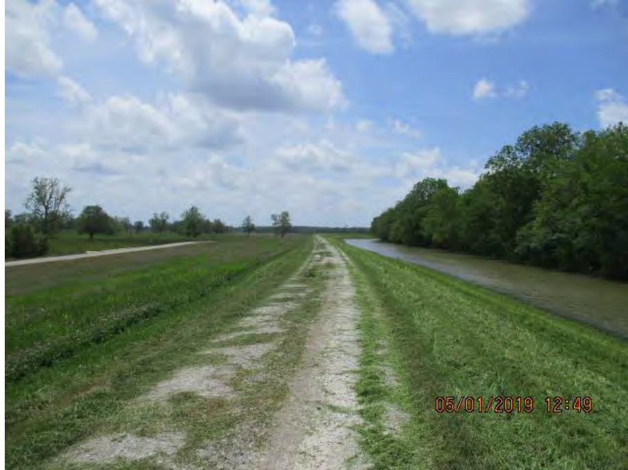
Figure 2: Southwest facing picture near the center of the alignment, Pointe Coupee Parish, Louisiana.
