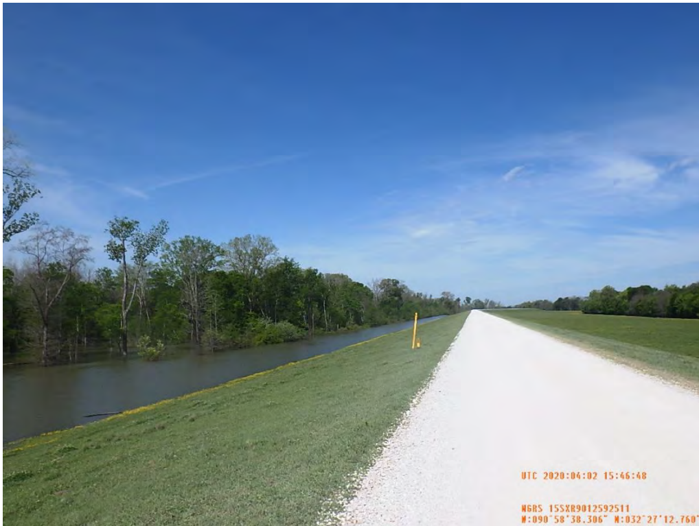
Figure 5: Northwest facing picture of the proposed levee enlargement, Warren County, Mississippi.
