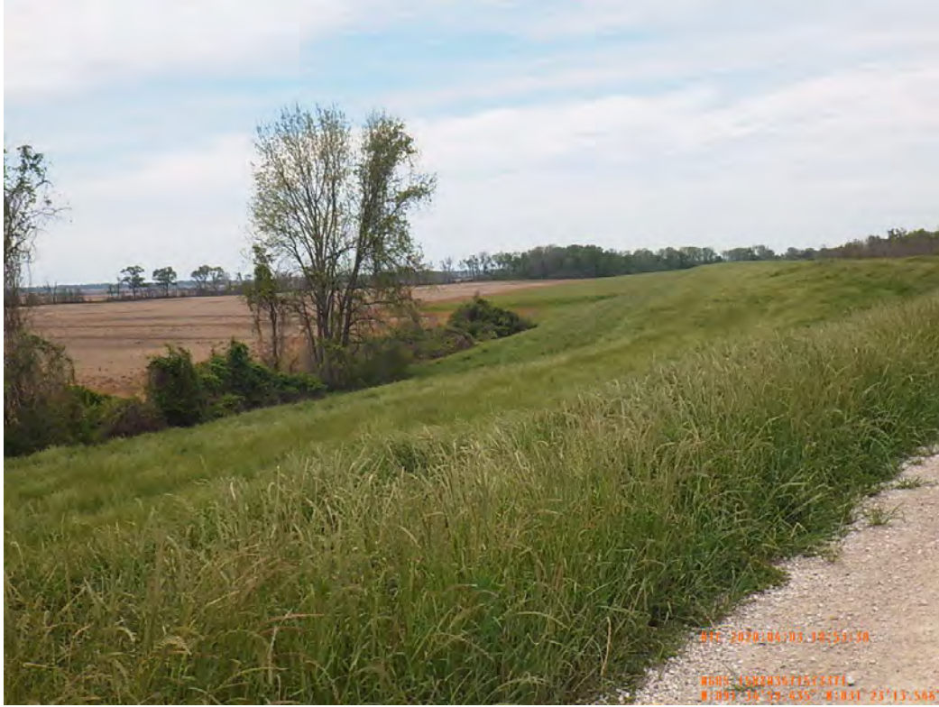
Figure 2: West facing picture for the proposed seepage berm, Concordia Parish, Louisiana.
