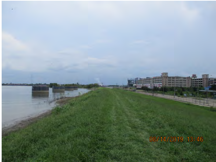
Figure 4: South facing picture near the center of the alignment_on west side of IHNC Forebay, Orleans Parish, Louisiana.
