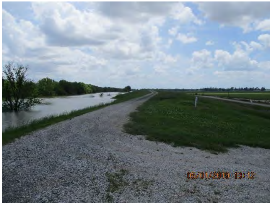
Figure 3: Southwest facing picture near the center of the alignment, West Baton Rouge Parish, Louisiana.
