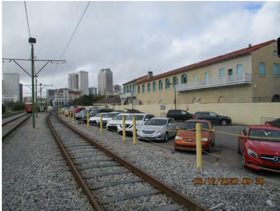
Figure 2: Southwest facing picture near the center of the alignment, Orleans Parish, Louisiana.
