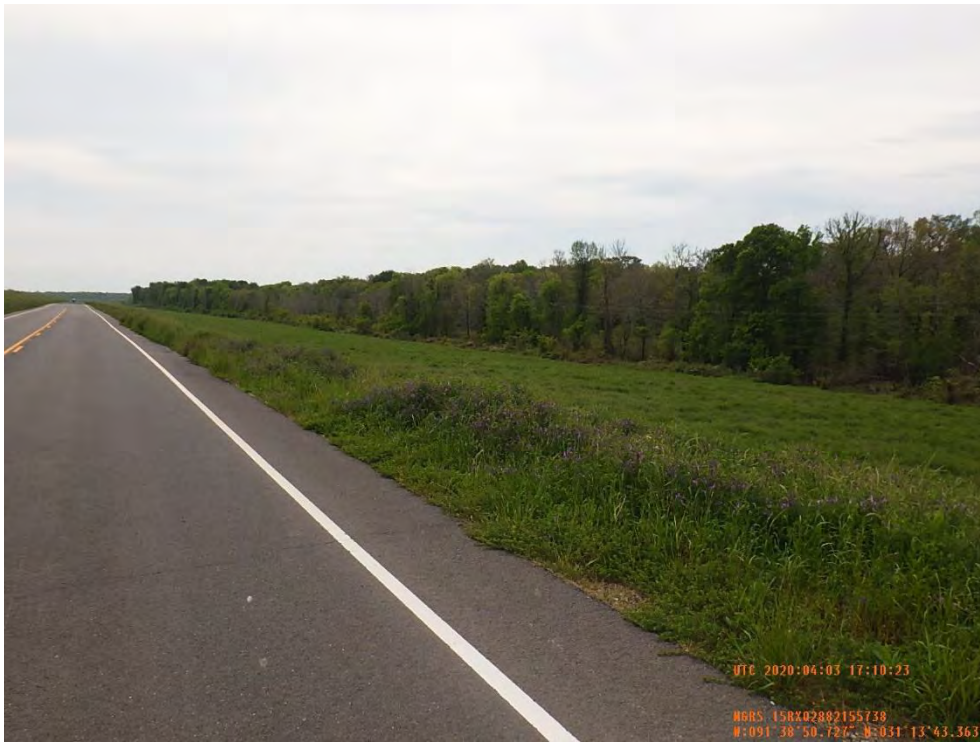
Figure 5: Southwest facing picture of levee toe for proposed seepage berm, Concordia Parish, Louisiana.
