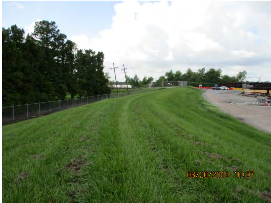
Figure 2: South facing picture on east side of the Chalmette Slip, St. Bernard Parish, Louisiana.
