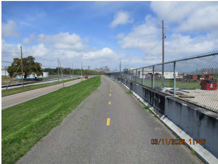
Figure 2: North facing picture near the center of Section 1 of the alignment, Jefferson Parish, Louisiana.
