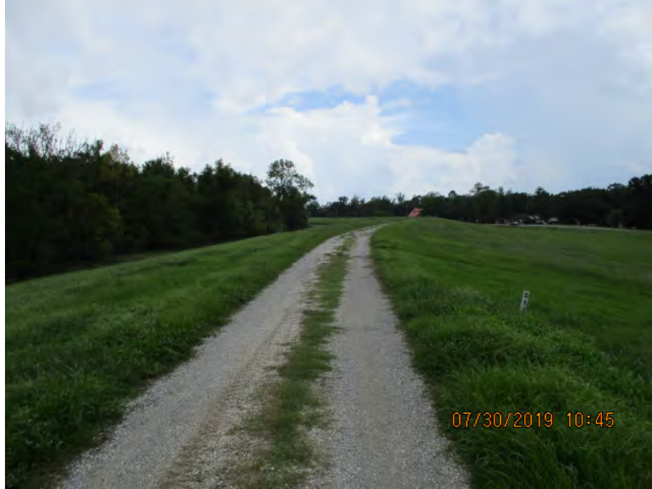
Figure 2: North facing picture near the center of the alignment, Saint Charles Parish, Louisiana.
