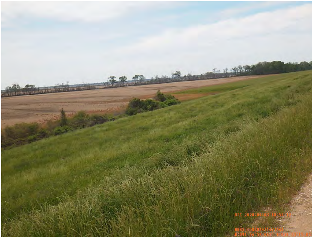
Figure 3: West facing picture for the proposed seepage berm, Concordia Parish, Louisiana.
