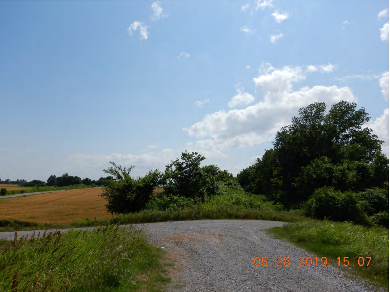
Figure 2: Representative photograph of the project area, facing downstream (southwest) along the levee.
