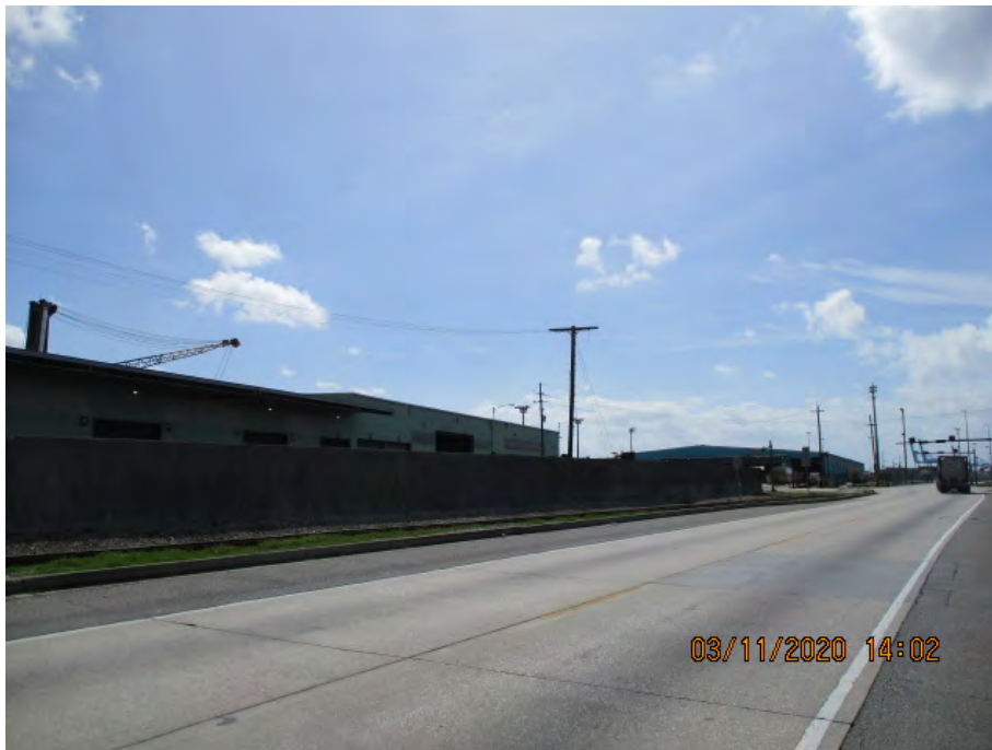
Figure 3: East facing picture near the center of the alignment, Orleans Parish, Louisiana.
