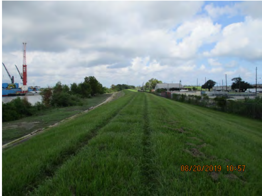
Figure 2: West facing picture near west end of the alignment, St. Bernard Parish, Louisiana.
