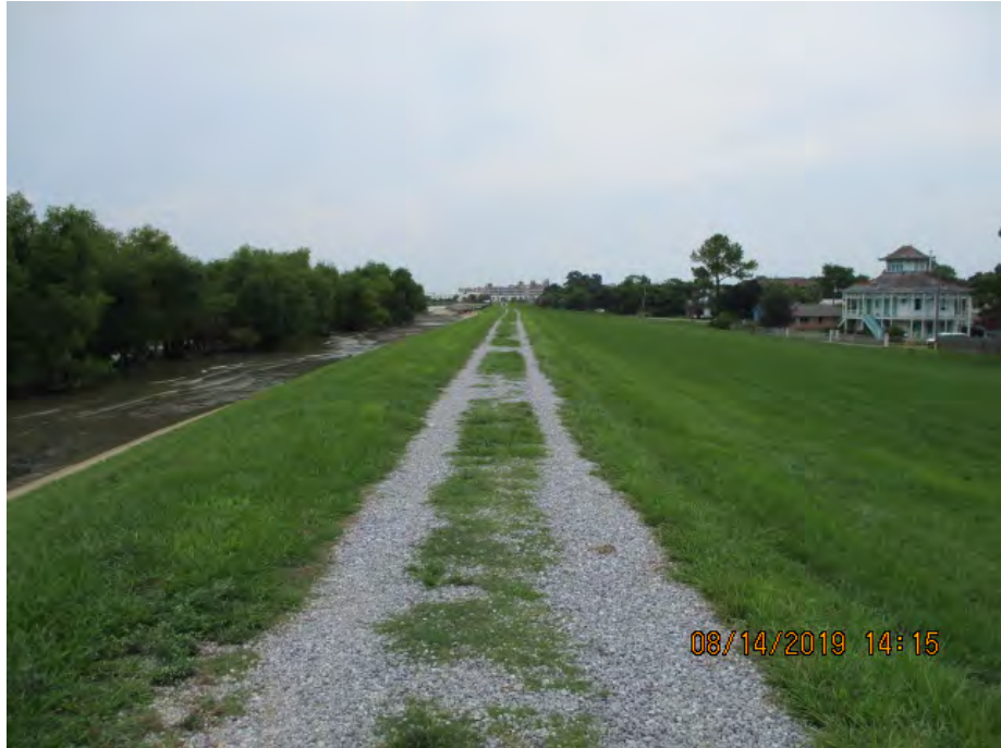
Figure 2: West facing picture near the center of the alignment, Orleans Parish, Louisiana.
