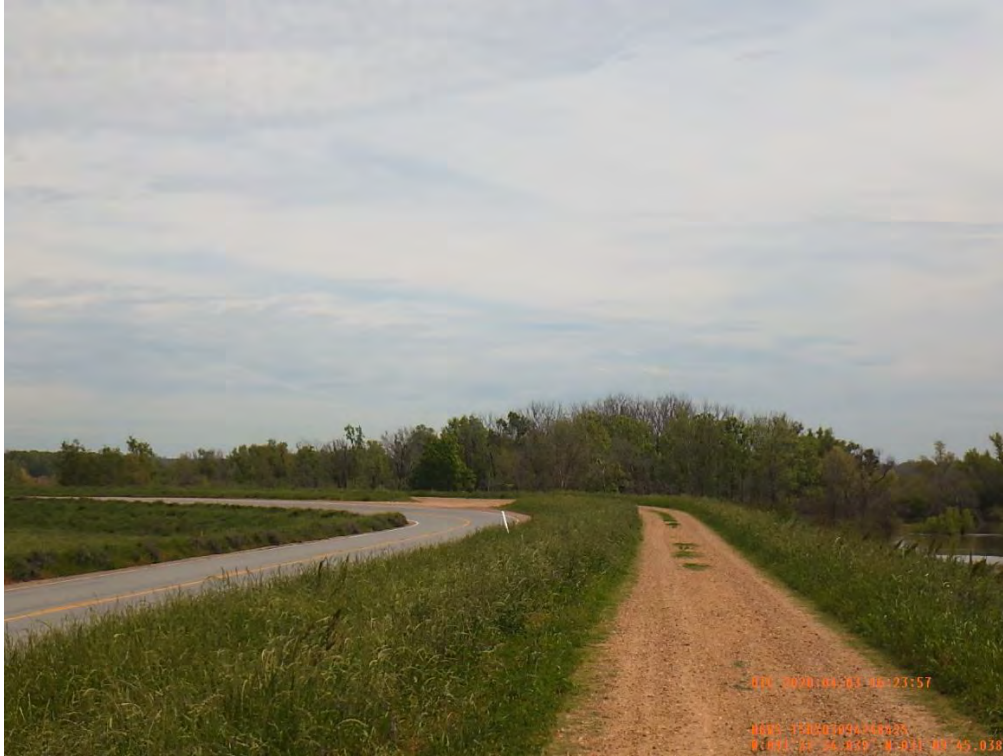
Figure 2: Northwest facing picture from the center of the alignment, Concordia Parish, Louisiana.
