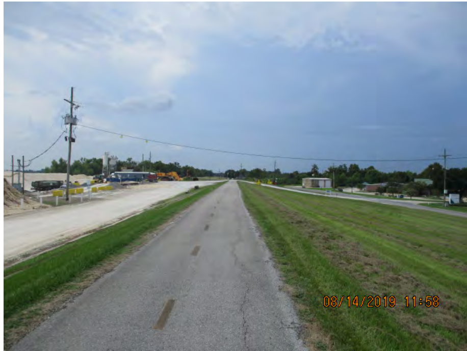
Figure 2: Southwest facing picture near the center of the alignment, St. Charles Parish, Louisiana.
