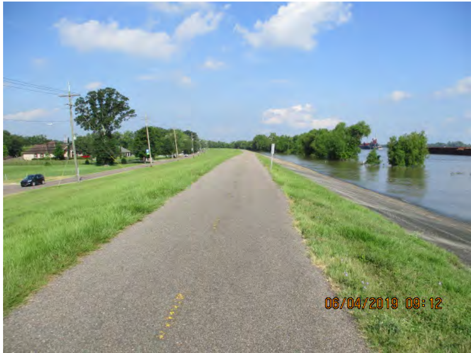
Figure 2: West facing picture near the center of the alignment, Jefferson Parish, Louisiana.
