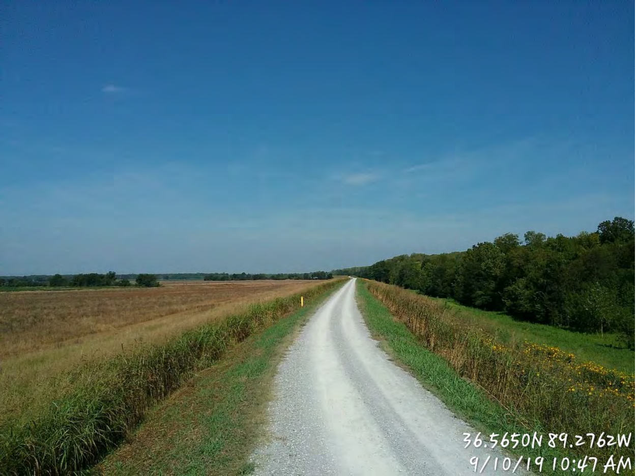
Figure 2: Representative photograph of the project area, facing downstream (southwest) along the levee within the project area. Proposed relief wells would be installed landside of the levee (left side of the photograph).
