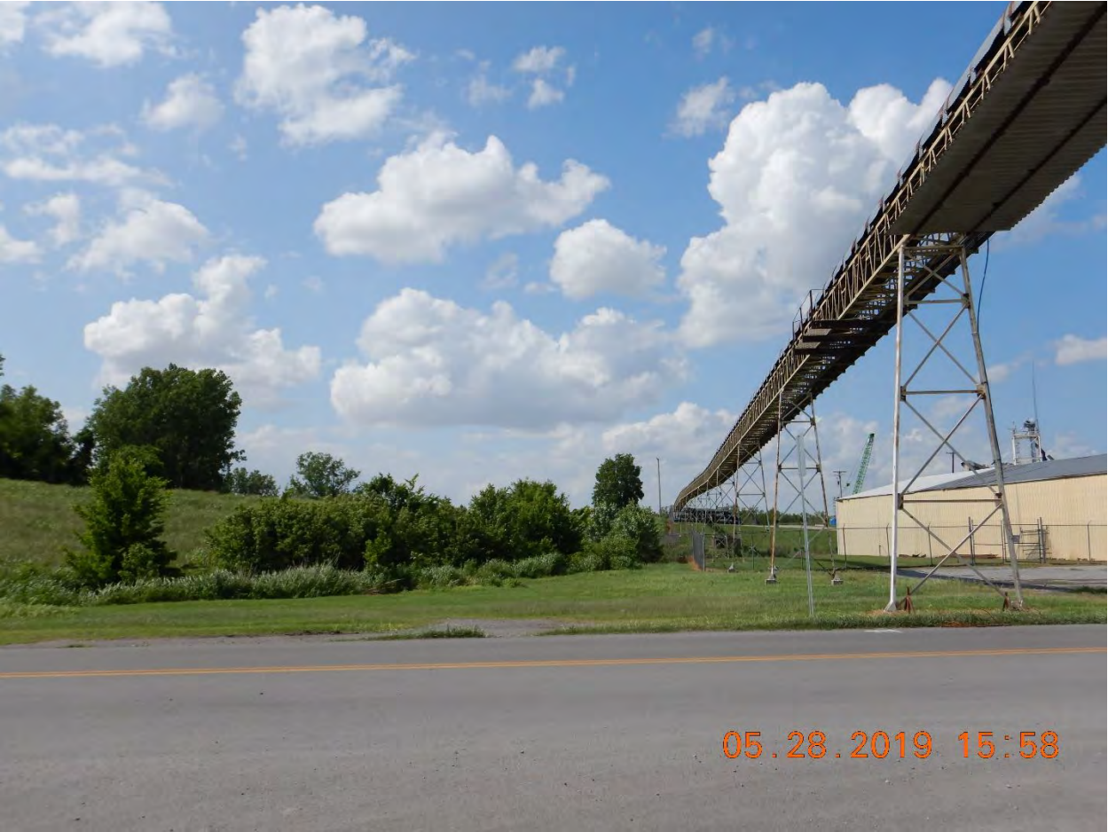
Figure 2: Representative photograph of the project area, facing the levee (north) from Catlett Street.
