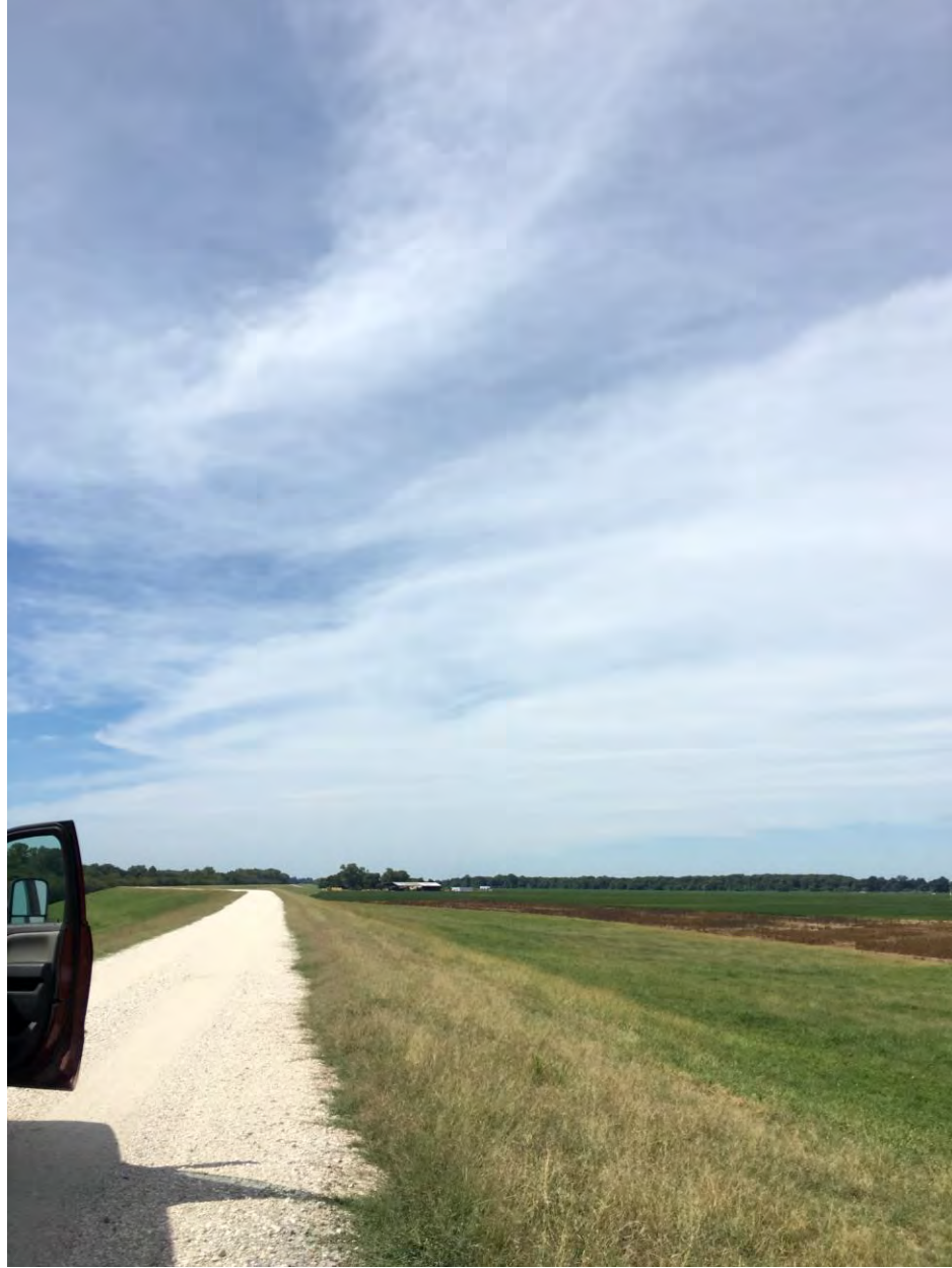
Figure 2: Representative photograph of the site, facing SW (downstream) along the mainline Mississippi River Levee crown near Clark Road or Levee Station 177/35+33 within the proposed project boundaries.
