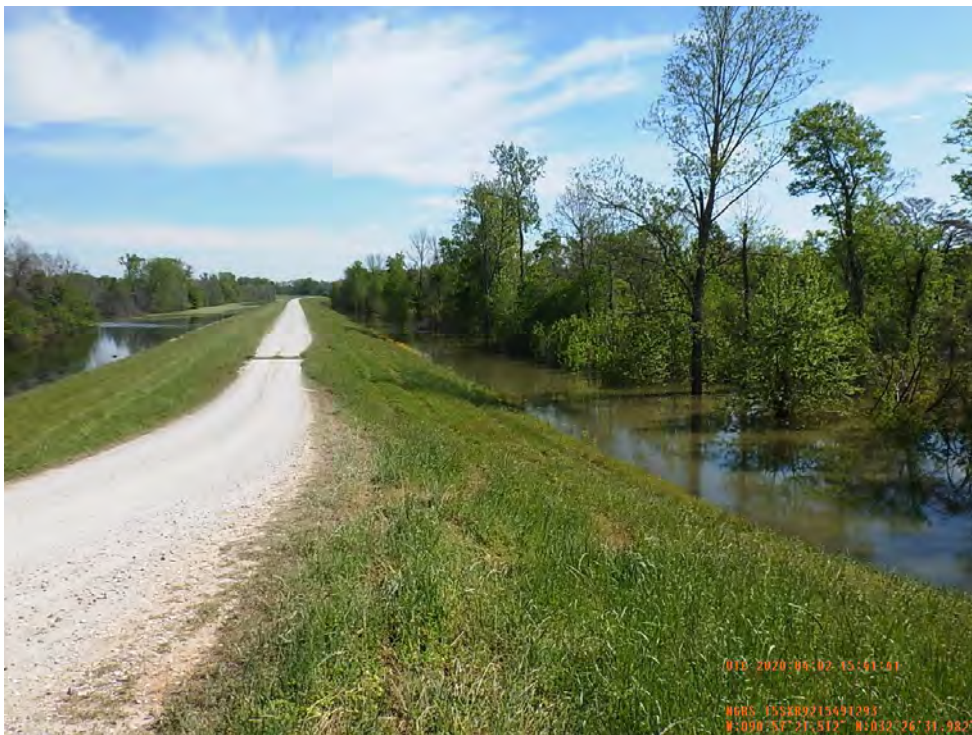
Figure 3: Southeast facing picture of the proposed levee enlargement, Issaquena County, Mississippi.
