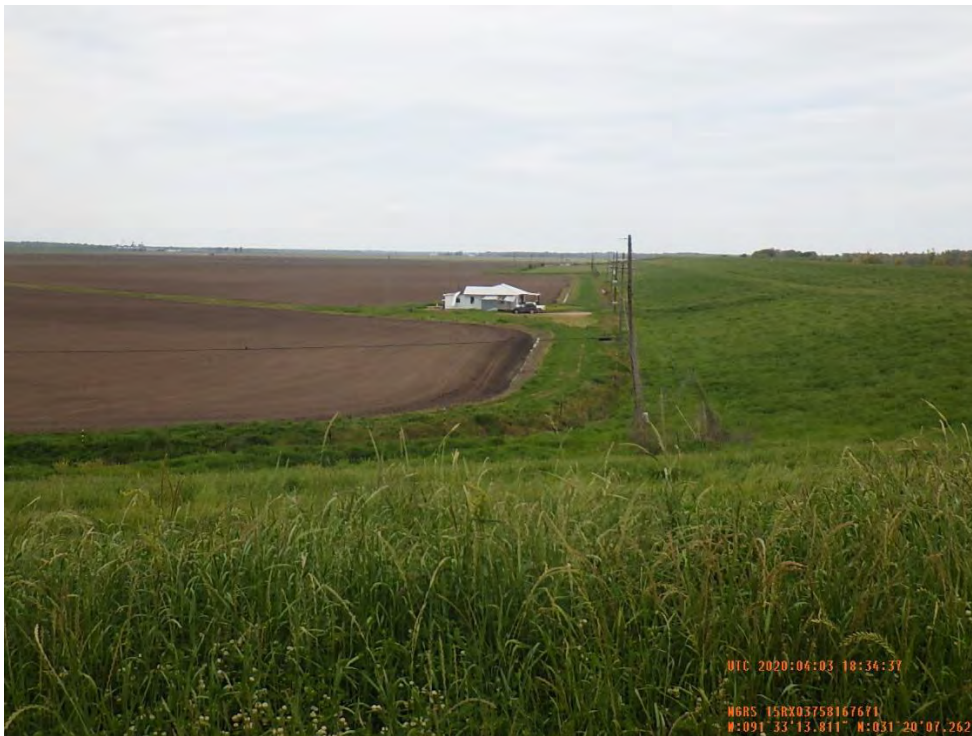
Figure 3: Northwest facing picture for the proposed location of seepage berm with residential structure, Concordia Parish, Louisiana.
