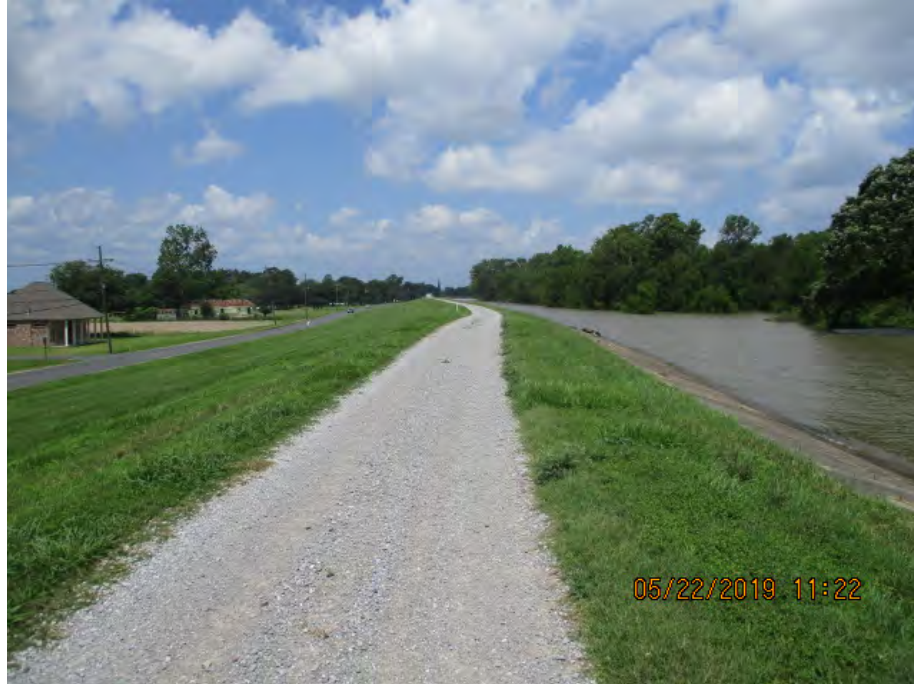
Figure 2: Northwest facing picture near the center of the alignment, Ascension Parish, Louisiana.
