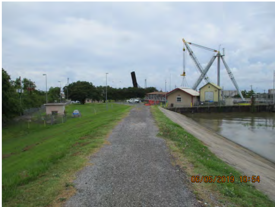
Figure 3: South facing picture near the center of the alignment, East side of the Harvey Canal, Jefferson Parish, Louisiana.
