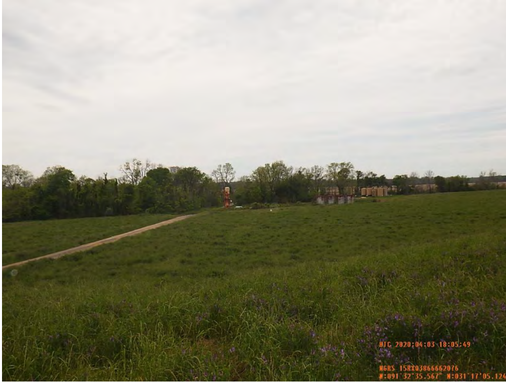
Figure 4: West facing picture of existing relief wells in the proposed location for future relief wells with petroleum tank farm excluded from string on existing wells, Concordia Parish, Louisiana.
