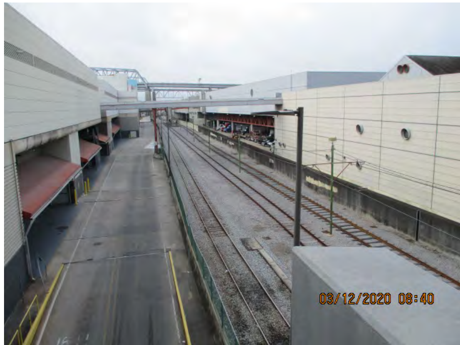
Figure 3: North facing picture near the center of the alignment, Orleans Parish, Louisiana.
