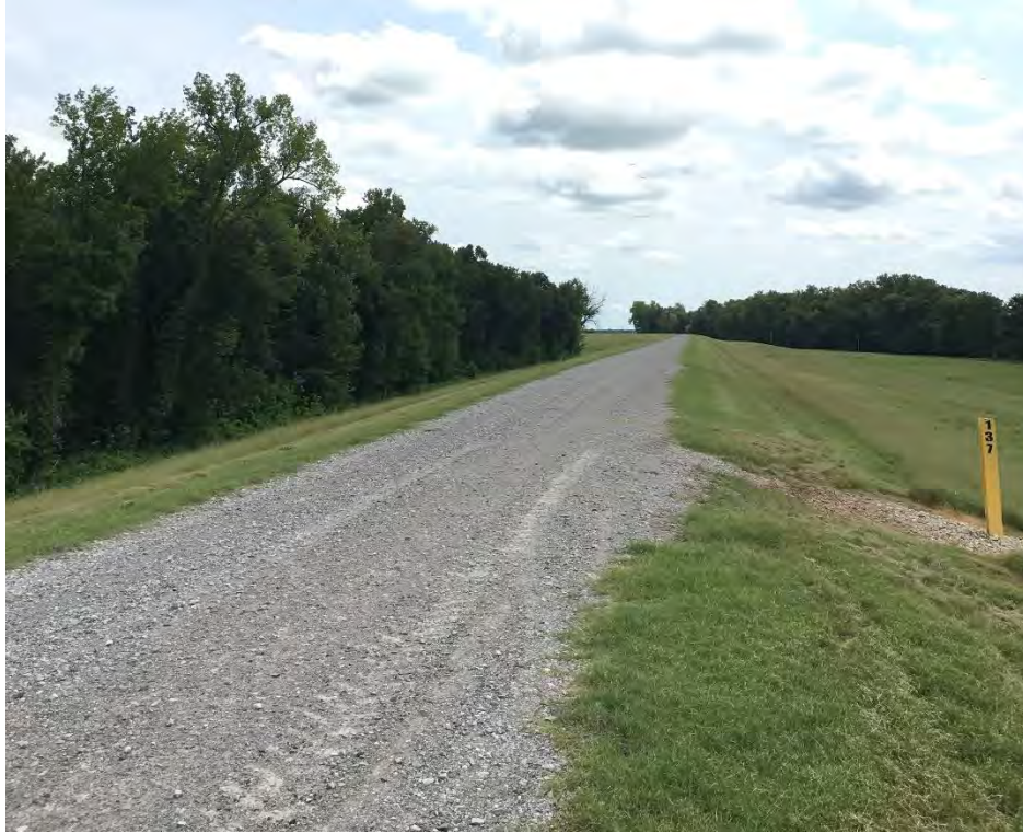
Figure 2: Representative photograph of the project area, facing downstream at Levee Station 137.
