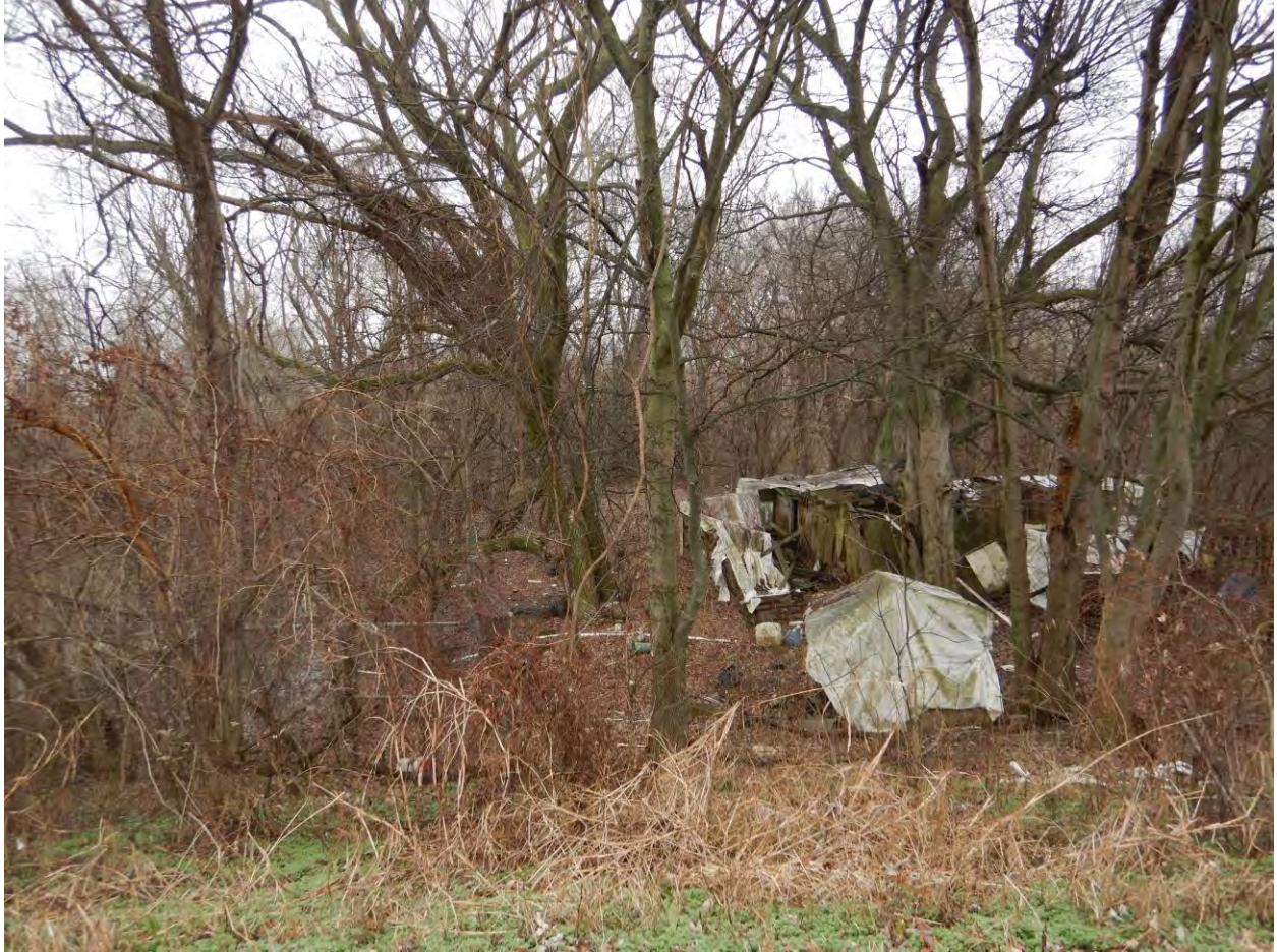
Figure 3: Photograph from levee facing riverside (south) near the old Fish Market, showing the area requiring further investigation during detailed design.
