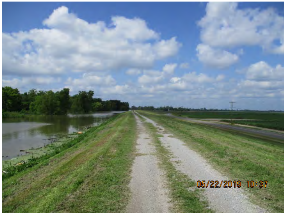
Figure 3: Southwest facing picture near the center of the alignment, Ascension Parish, Louisiana.
