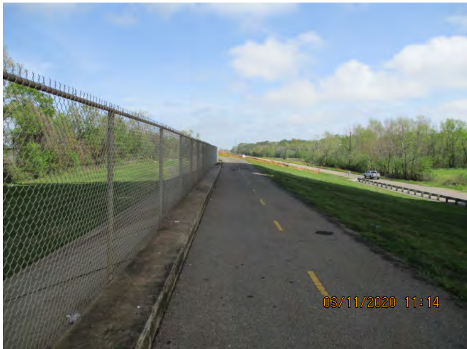
Figure 5: Northeast facing picture near the center of the Bridge City Floodwall alignment, Jefferson Parish, Louisiana
