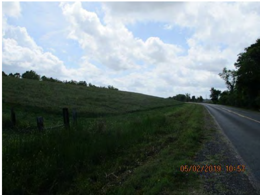
Figure 3: Southeast facing picture near the center of the alignment, West Baton Rouge Parish, Louisiana.
