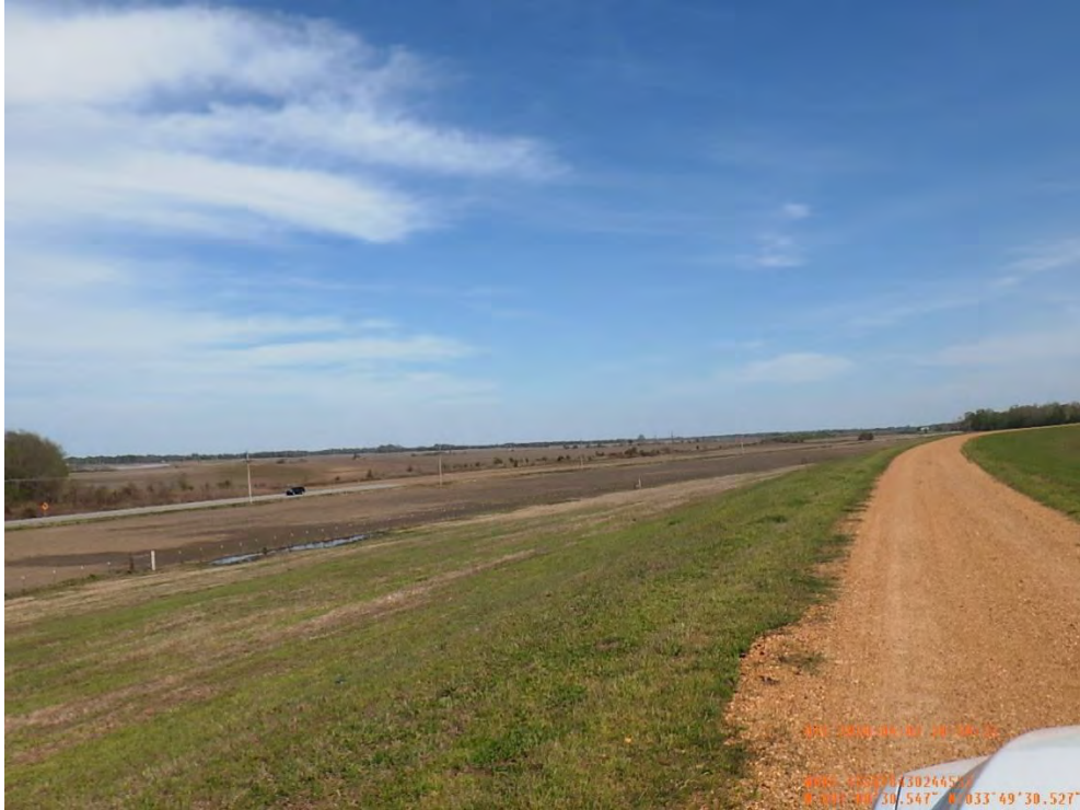
Figure 4: Southeast facing picture of the proposed seepage berm location, Bolivar County, Mississippi.
