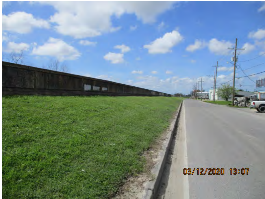
Figure 2: Northwest facing picture near the center of the alignment, St. Bernard Parish, Louisiana.
