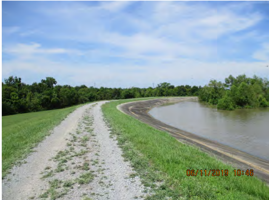
Figure 5: Southwest facing picture near the center of the alignment, Orleans Parish, Louisiana.
