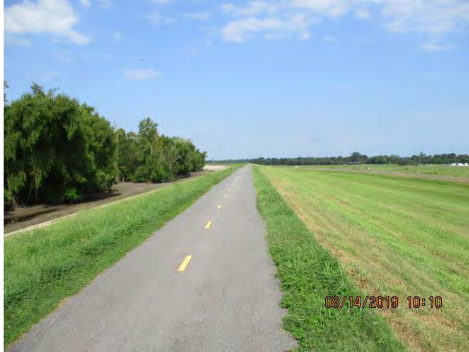
Figure 2: Northwest facing picture near the center of the alignment, East Baton Rouge Parish, Louisiana.
