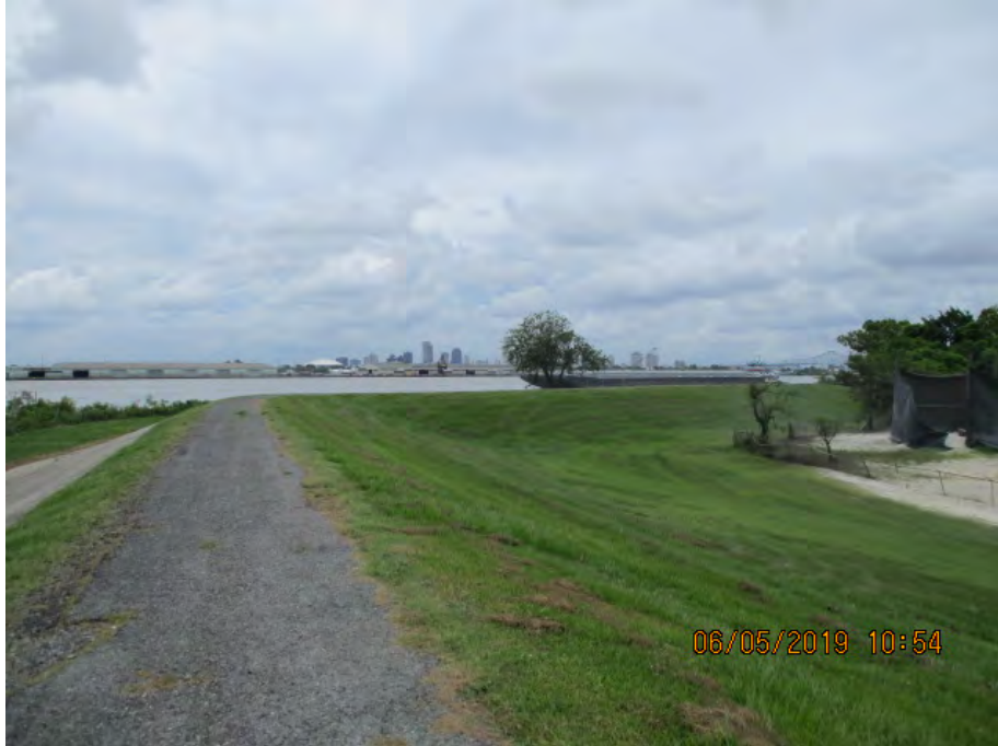
Figure 2: North facing picture near the center of the alignment, East side of the Harvey Canal, Jefferson Parish, Louisiana.
