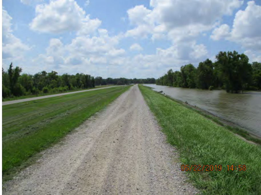
Figure 2: Northwest facing picture near the center of the alignment, Saint James Parish, Louisiana.
