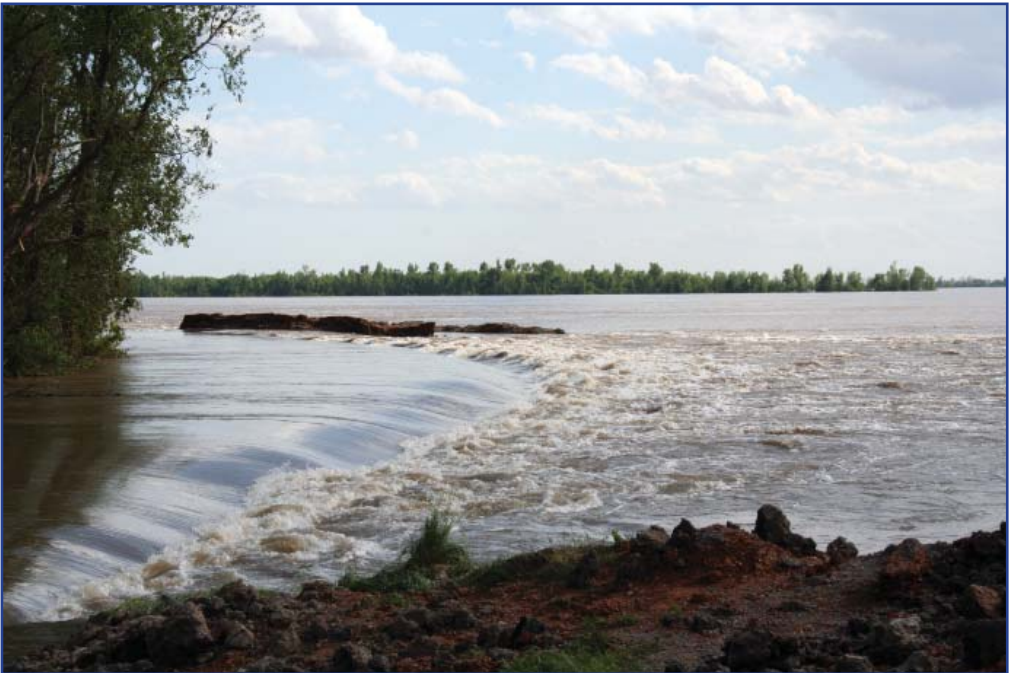
Water roars through the upper inflow crevasse at the frontline levee the day after activation.
