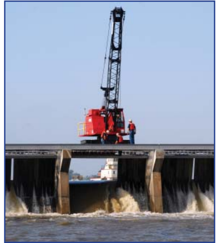
Raising the needles at the Bonnet Carré spillway.
