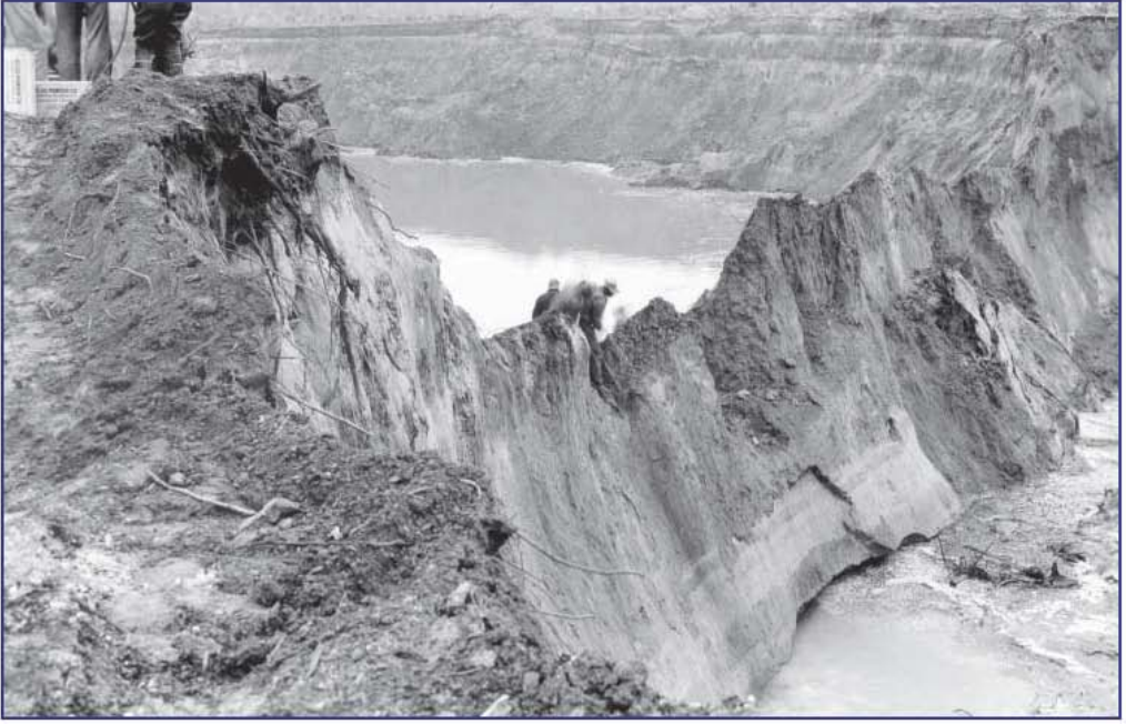
An earthen plug is all that separates the dredged pilot channels.
