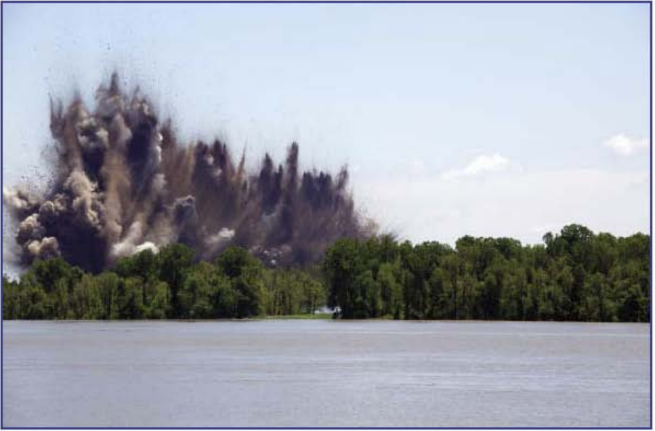
Above: Activation of the lower inflow/outflow crevasse site on May 3, 2011. Below: Aerial view of the upper crevasse site after activation of the floodway.
