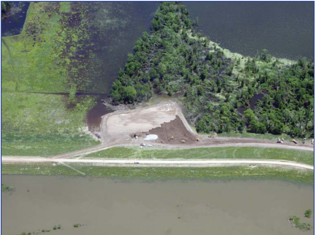
The hired-labor crew begins placing the clay cap over the sand fill as water from Eagle Lake climbs higher against the earthen berm.
