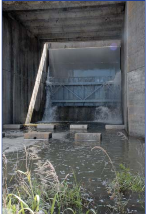
Water spills over the gates at the Morganza spillway.
