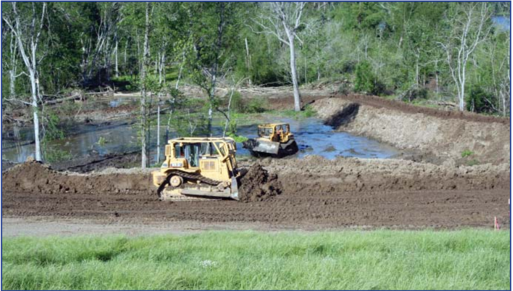
Hired-labor crews construct the earthen berm around Buck Chute, while continuing to clear the area.
