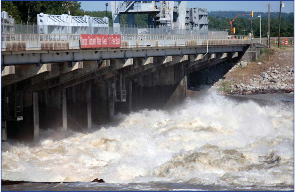
The Low Sill Structure at the Old River Control Complex on May 14, 2011.
