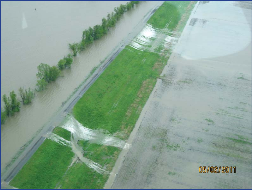
Passive activation of the floodway. The Mississippi River overtops the lower sections of the Birds Point-New Madrid floodway fuseplug levee early on May 2, 2011.
