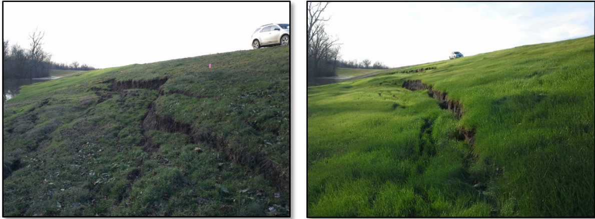
Figure 1-4. Profile and photographs showing levee slides in need of slope flattening.
