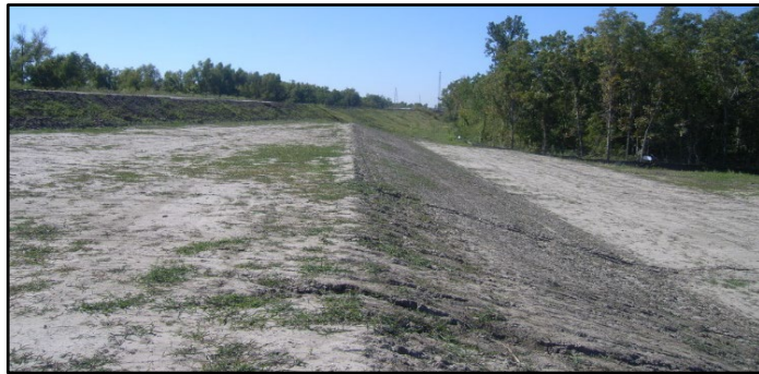
Figure 1-5. Profile and photographs of a typical seepage berm along the MRL.
