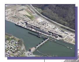
The 1200-foot locks can accommodate a tow of 17 barges plus the towboat, while the 600-foot locks can accommodate at most eight barges plus the towboat. The lock size and tow size are critical factors in the amount of cargo that can pass through a lock in a given period of time. Since many of today's tows operate with 12 or more barges,
